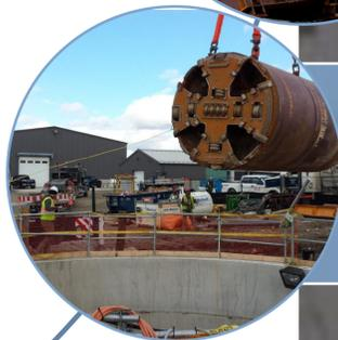
The selected tunnel boring machine(s) will be equipped to handle known deep, water-bearing buried valley geohazards which have slowed similar projects in the area.
