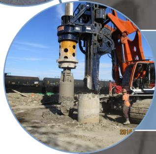
Surface impacts limited to shaft and working compound construction. Shafts provide launch and reception locations for the specialized tunnel boring machines.
