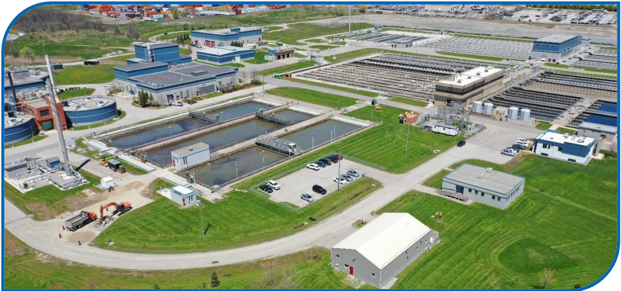
Figure 8 – Clarkson Wastewater Treatment Plant.
