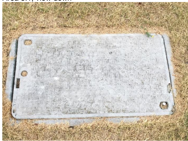
Photo 22: Buried utilities located throughout Area 5.1; view down
