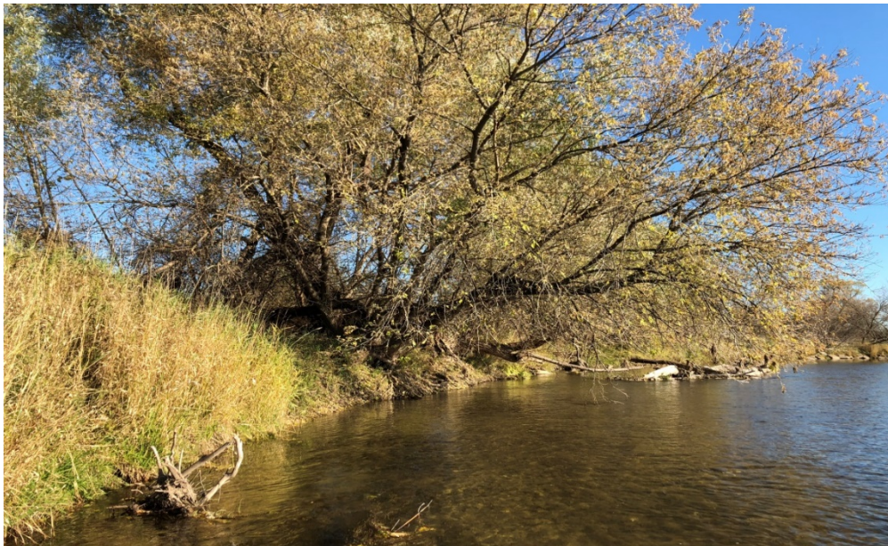
Photograph 2: Reach CR-1; exposed tree roots and leaning trees over channel, as well as abundant woody debris within channel.
