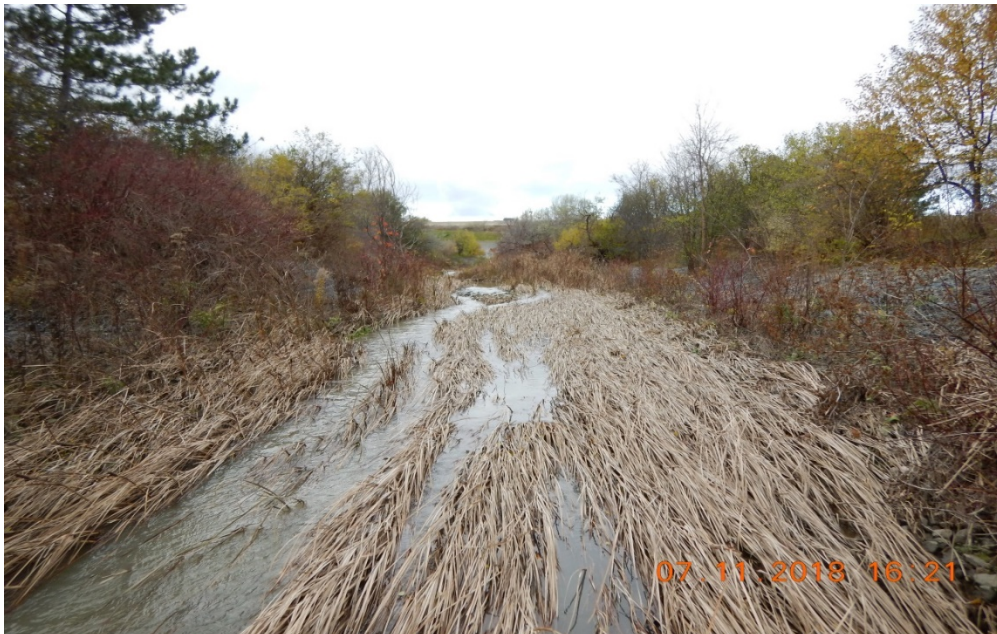
Photograph 10: Reach MC-1; view upstream of Century Ave.; abundant instream growth of tall grass, banks are lined with sloped gabion baskets.
