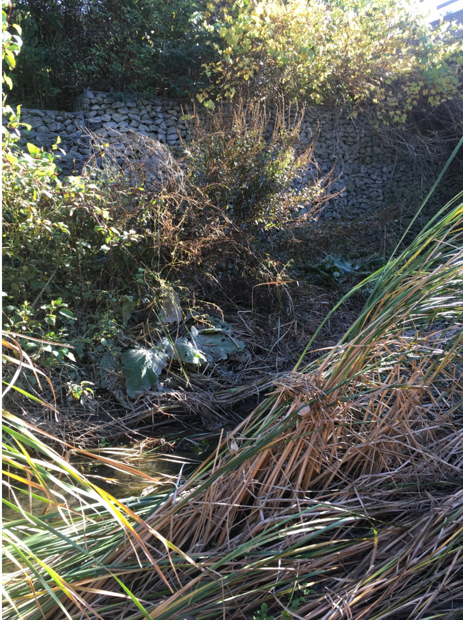
8. View of gabion baskets along bank of Mullet Creek downstream of Highway 401 at Site 8.
