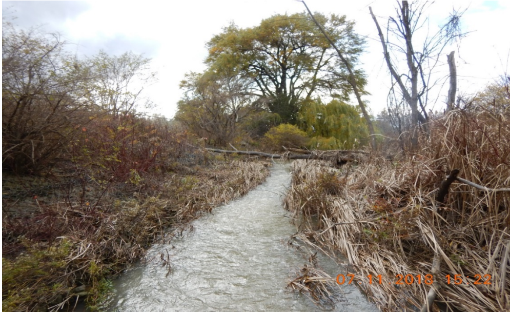
Photograph 3: Reach MC-1; view upstream with highway 401 along right bank (left side of photo); there is a fallen down tree across the channel and the banks remain lines with gabion baskets.
