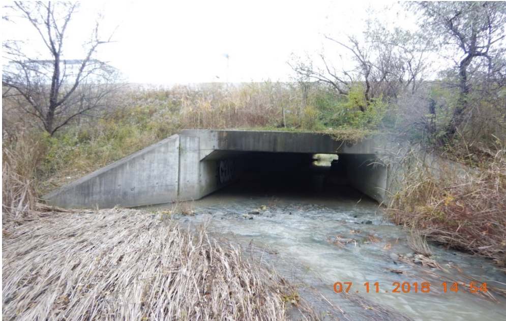
Photograph 5: Reach MC-1; looking downstream at bridge crossing with Highway 401 (on upstream side); tall grass within channel and cobble-sized sediment at culvert opening.
