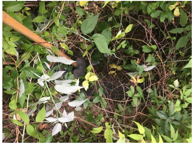
Photo 10: Culvert located within Area 4.2; view down
