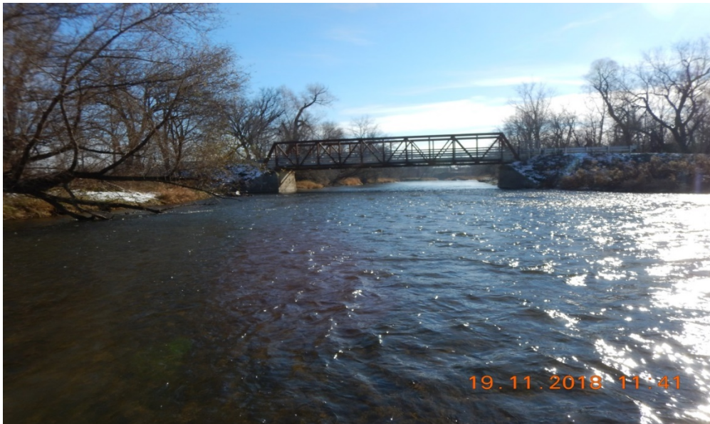
Photograph 20: Reach CR-2; downstream extent of reach towards crossing with pedestrian bridge.
