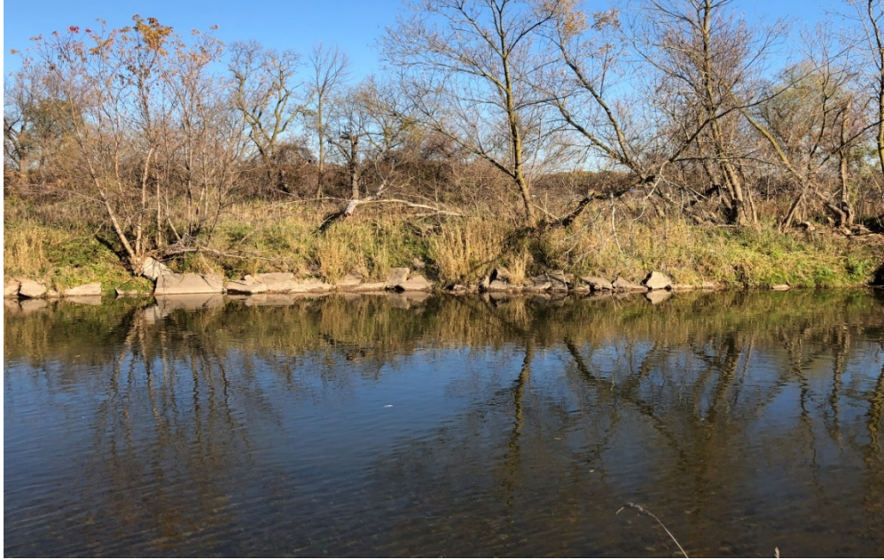
Photograph 3: Reach CR-1; large slabs of concrete (up to ~1.5 m in length) that have washed up along the left bank from further upstream.
