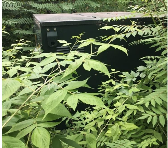
Photo 12: Utility box found within Area 4.2; view west
