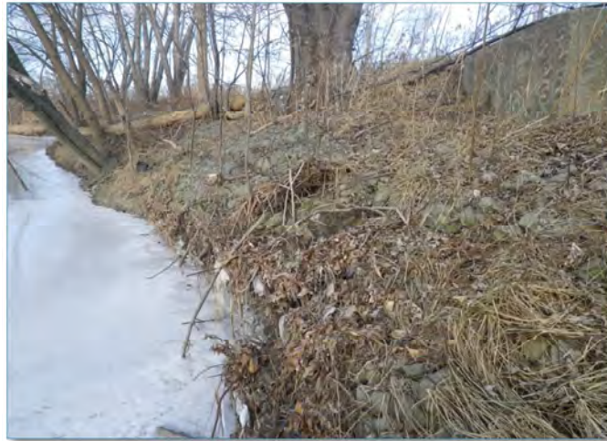
Figure 3: Manhole Protected by Gabion along Right Bank of Cooksville Creek.
