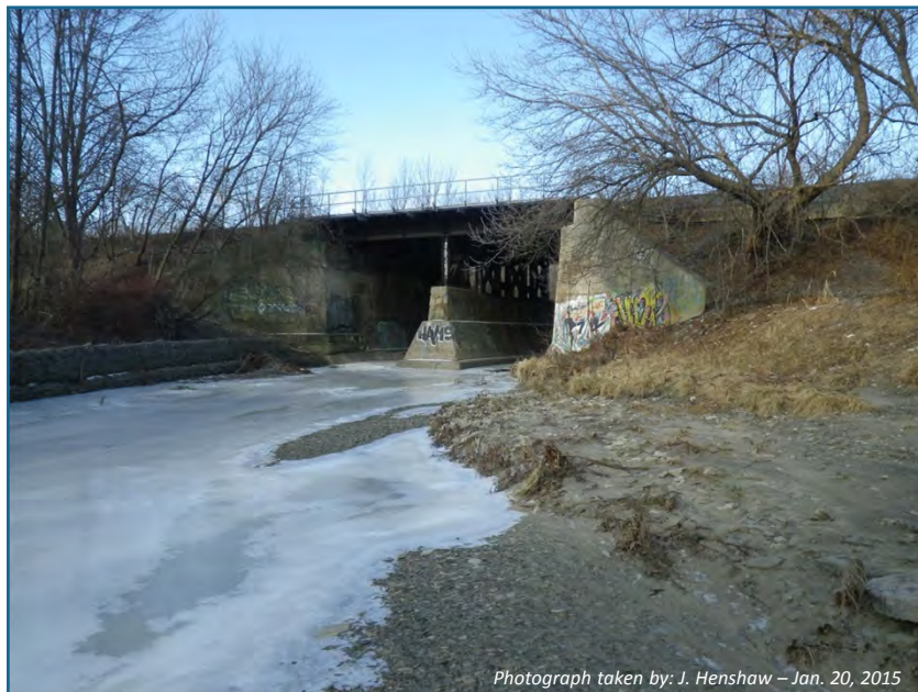
Photograph taken by: J. Henshaw – Jan. 20, 2015
