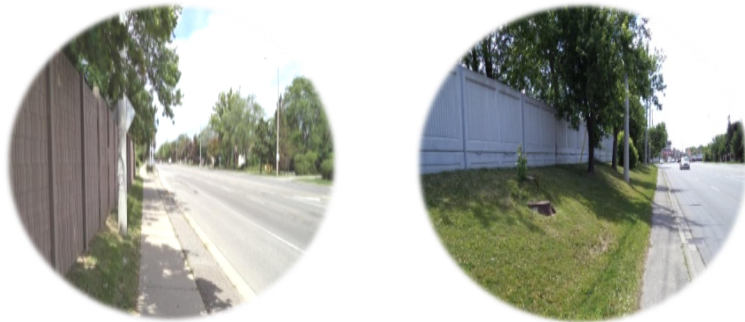
Existing Noise Walls
