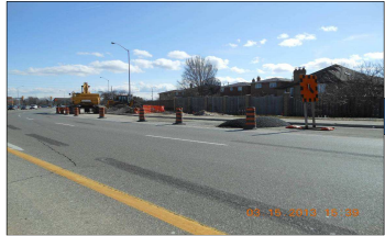
Burnhamthorpe Intersection Improvements
