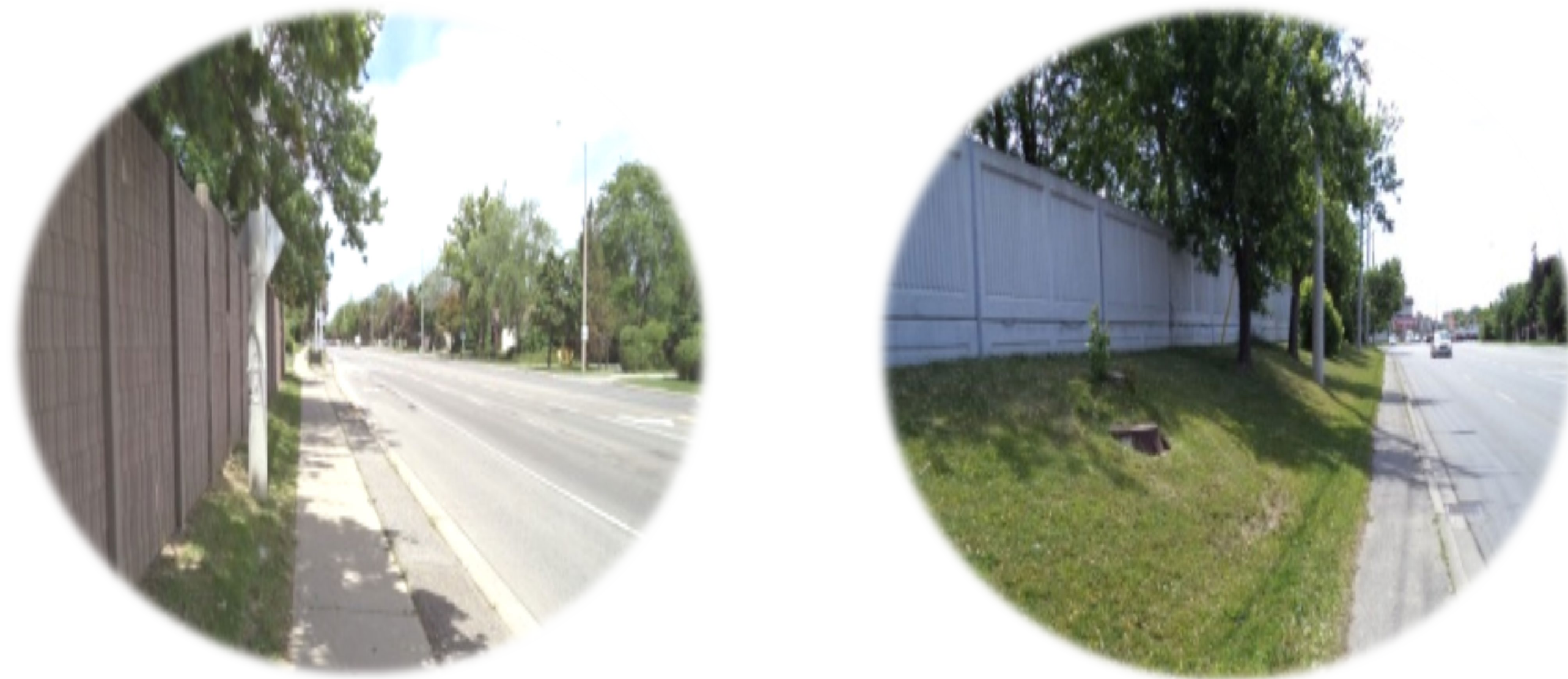
Existing Noise Walls
