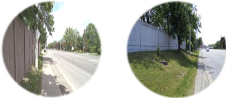
Existing Noise Walls
