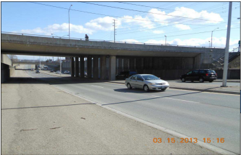
Dundas St and CP Railway Overpasses
