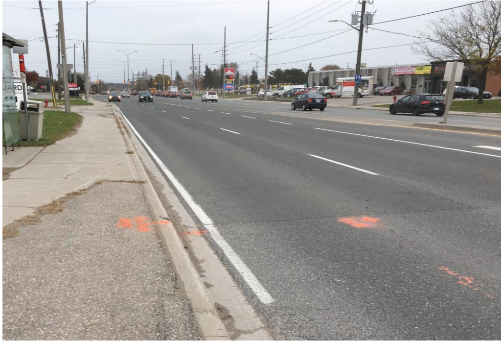
Photo 3: Cawthra Road at Sta. 11+340, Looking North
