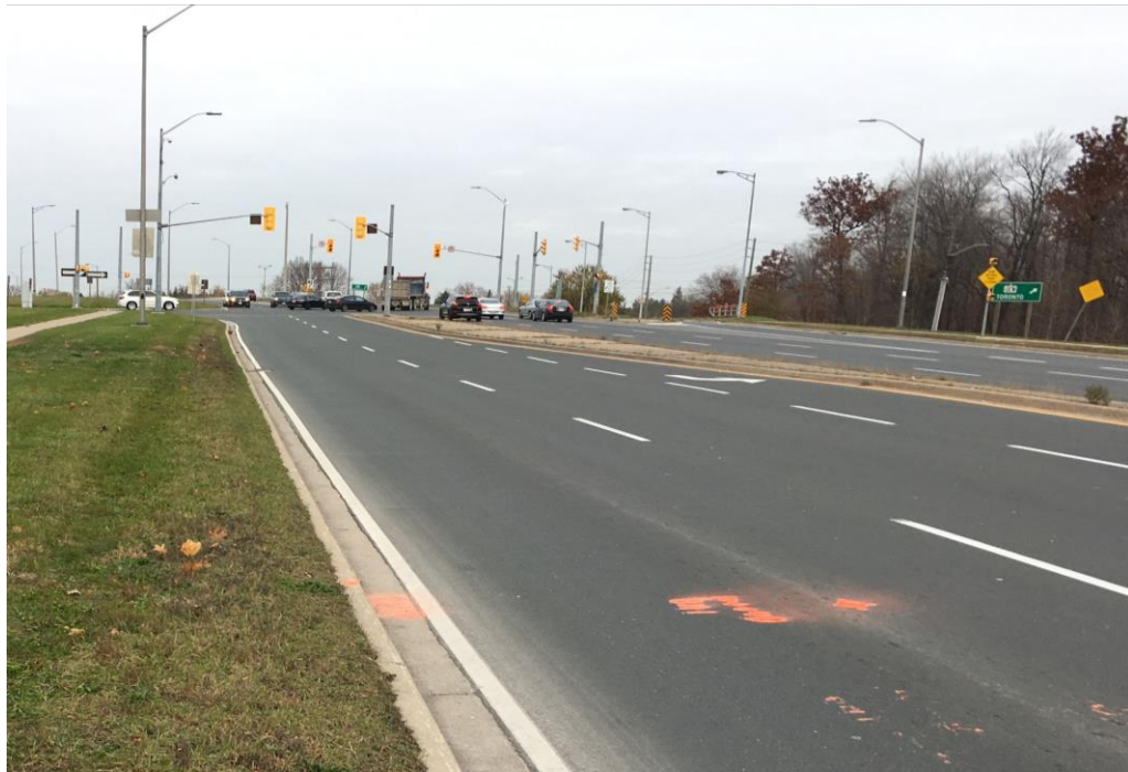
Photo 1: Cawthra Road at Sta. 10+040, Looking North
