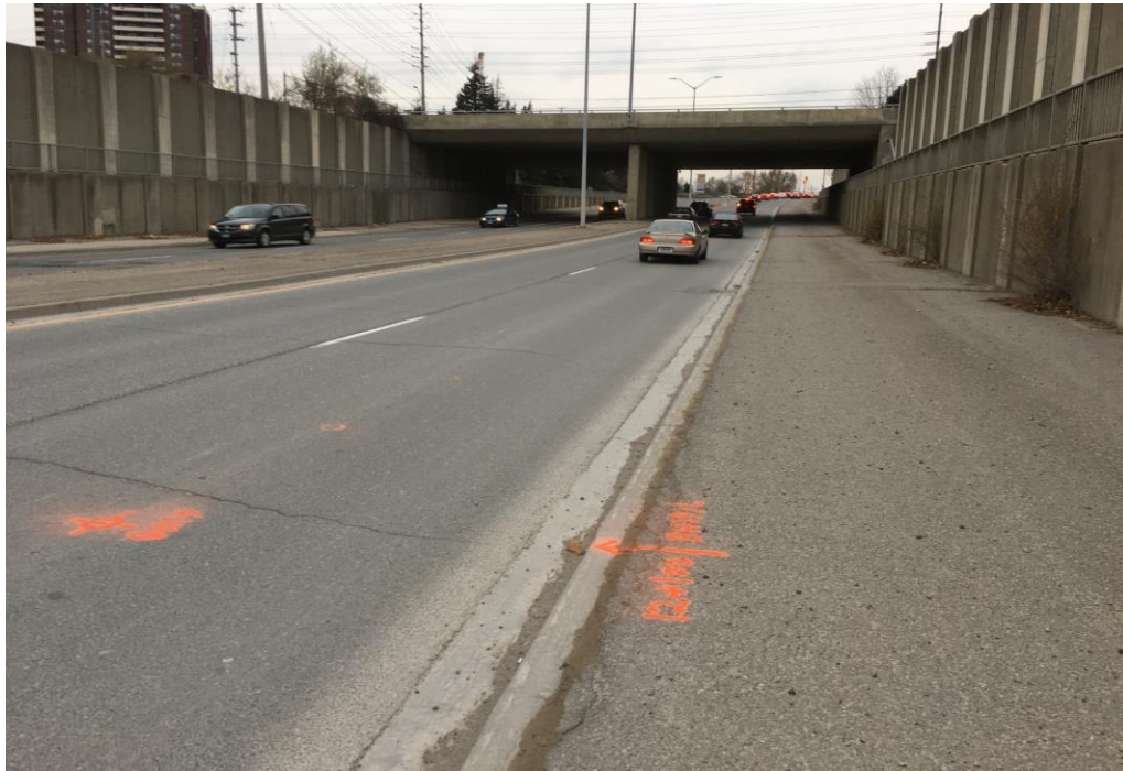
Photo 5: Cawthra Road at Sta. 12+100, Looking North
