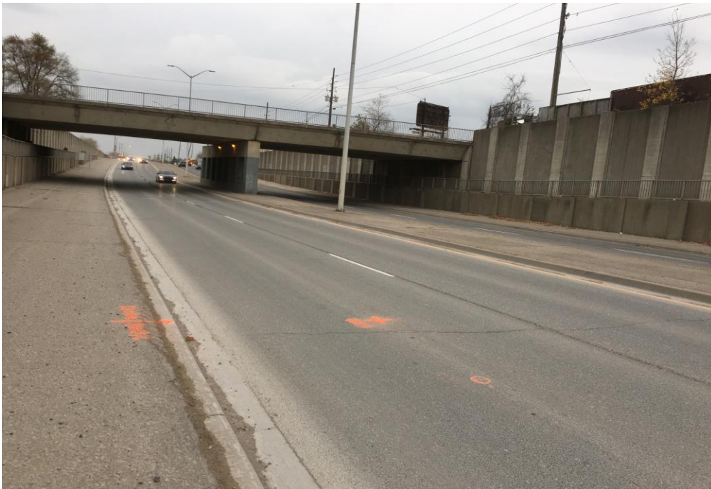
Photo 6: Cawthra Road at Sta. 12+100, Looking South
