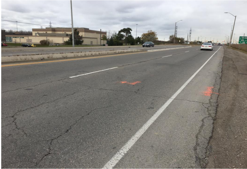
Photo 11: Cawthra Road at Sta. 15+110, Looking North
