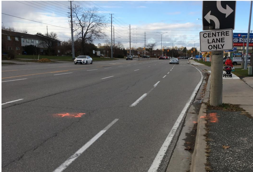
Photo 9: Cawthra Road at Sta. 14+100, Looking North
