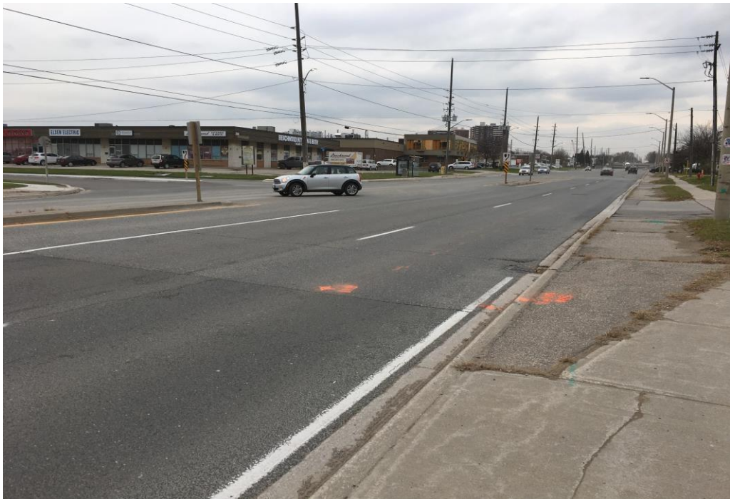
Photo 4: Cawthra Road at Sta. 11+340, Looking South
