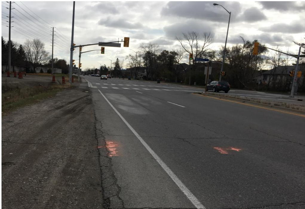
Photo 12: Cawthra Road at Sta. 15+110, Looking South
