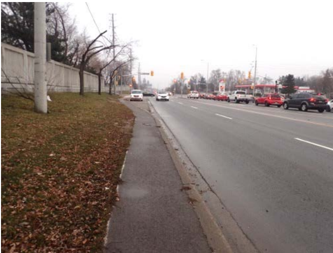
Image 27: View of paved roadway, curb, cut slope and grassed margin along the east side of Cawthra Road, north of Rathburn Road East.
