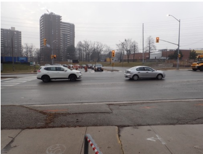
Image 11: View of paved roadway, pedestrian sidewalks, traffic island, cut slopes and graded margins, and utility installations at the junction of Dundas Street link and Cawthra Road.
