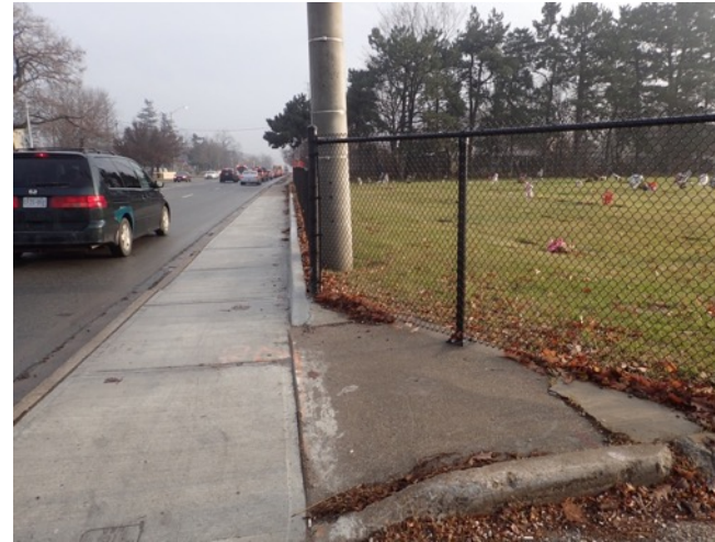
Image 18: View of paved roadway, sidewalk and hydro pole along the north (Cawthra Road-facing) margin of Mount Peace Roman Catholic Cemetery.
