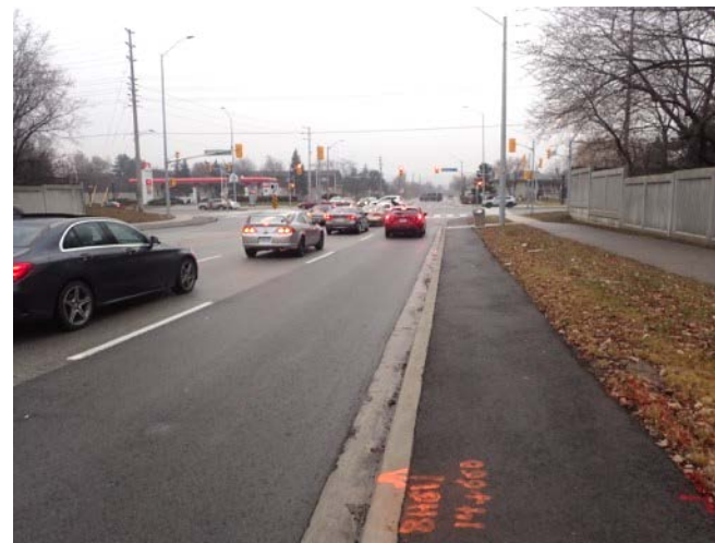
Image 26: View of paved roadway, curb, pedestrian sidewalks, utility installations and grassed margins along the north side of Rathburn Road East, east of Cawthra Road.
