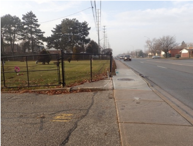
Image 17: View of paved roadway, sidewalk and manhole cover immediately outside, and paved access driveway to, the Mount Peace Roman Catholic Cemetery property.
