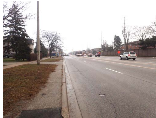
Image 22: View of paved roadway, curb, driveways, sidewalk, utility installations and testable grass frontages (beyond the sidewalk) along the east side of Cawthra Road, north of Bloor Street.
