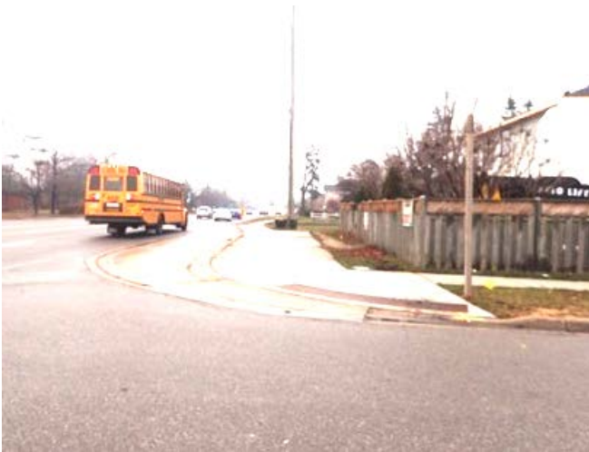
Image 25: View of paved roadway, pedestrian sidewalks, grassed margins and utility installations along west side of Cawthra Road, south of Hassall Road.
