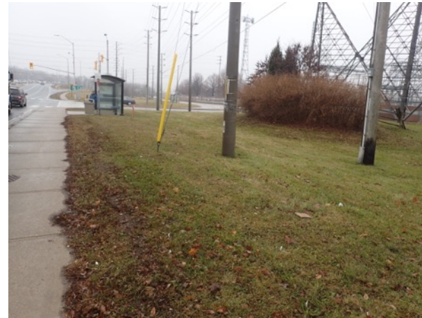
Image 4: View of pedestrian sidewalk, grassed margins, bus stop shelter and utility installations along the west side of Cawthra Road, north of North Service Road.
