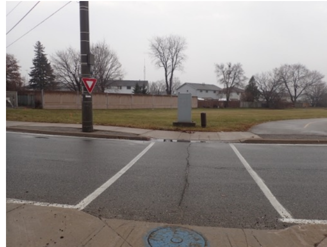
Image 6: View of paved roadway, traffic island, bike path, grassed margins, and utility installations at the southwest corner of the Cawthra Road-Queensway East intersection.
