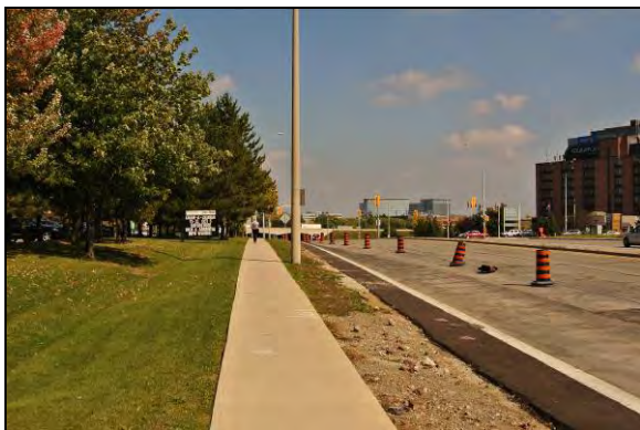
Plate 7: View northeast towards the intersection of Derry Road and Argentia Road
