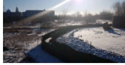
Floodplain Protection Measures
