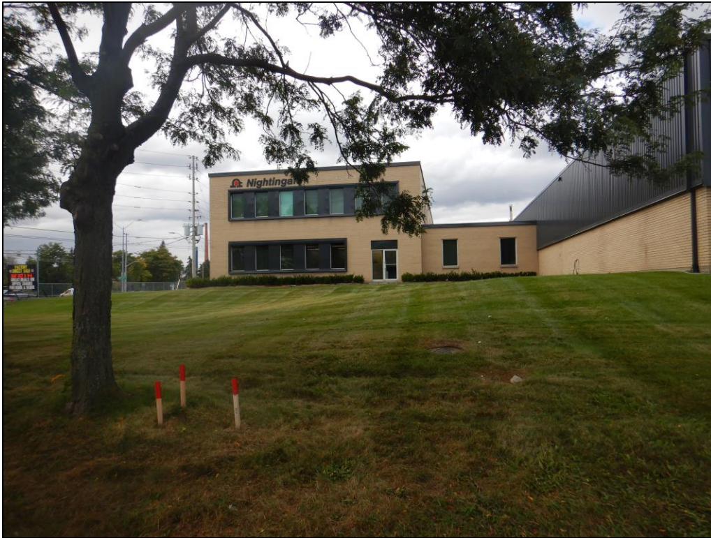
Photograph 5: Site 03A, looking northwest towards on-site manufacturing building.
