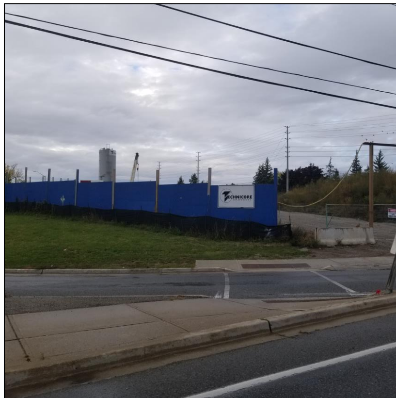
Photograph 20: Site 14B looking north
