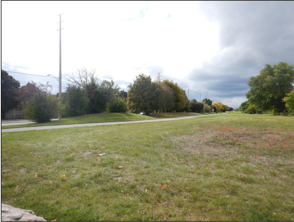
Photograph 11: Site 08B looking southwest.
