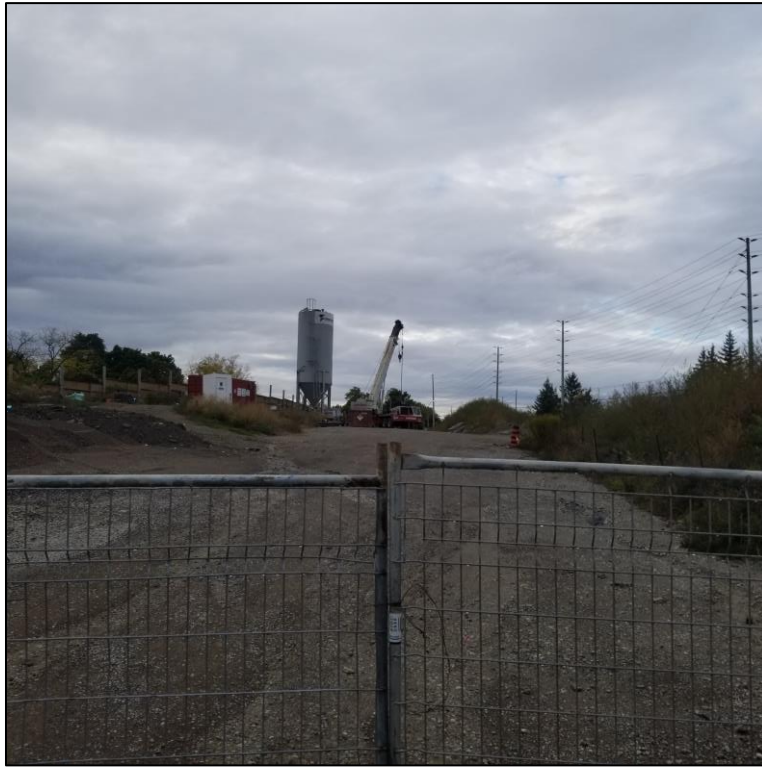
Photograph 21: Site 14B looking north.
