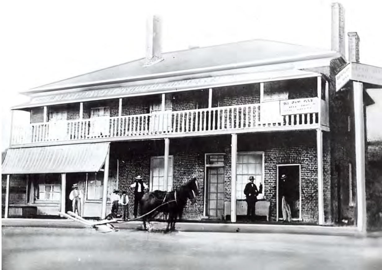
Figure 4: Atlantic Hotel in Dixie, date unknown (City of Mississauga 2020)
