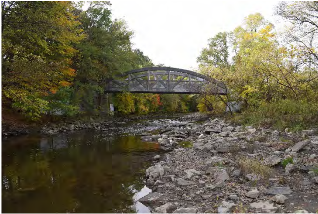
Middle Road Bridge, facing northwest from Etobicoke Creek
