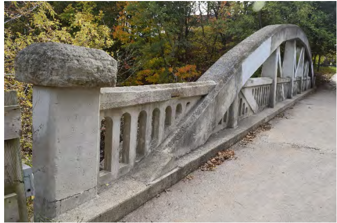
South side of Middle Road Bridge from bridge crossing
