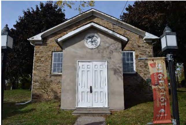
Southern entrance, facing north
