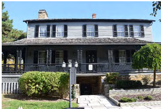
South west façade
