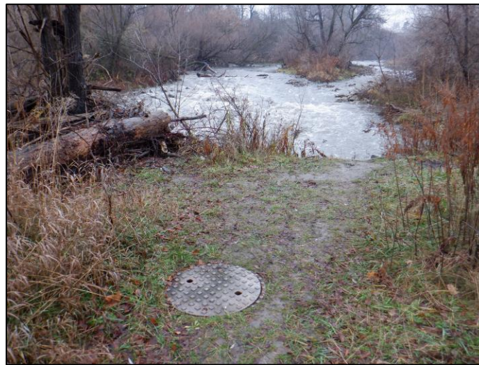
Image 2. Manhole within Area A facing southwest.
