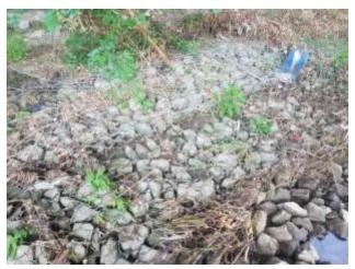
Photo 2: Gabion Basket erosion protection on the west bank at Queensway Bridge
