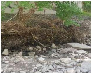
Photo 10: Undercut gabion basket at Sherway Drive Bridge (east side), downstream of Cross Section 3
