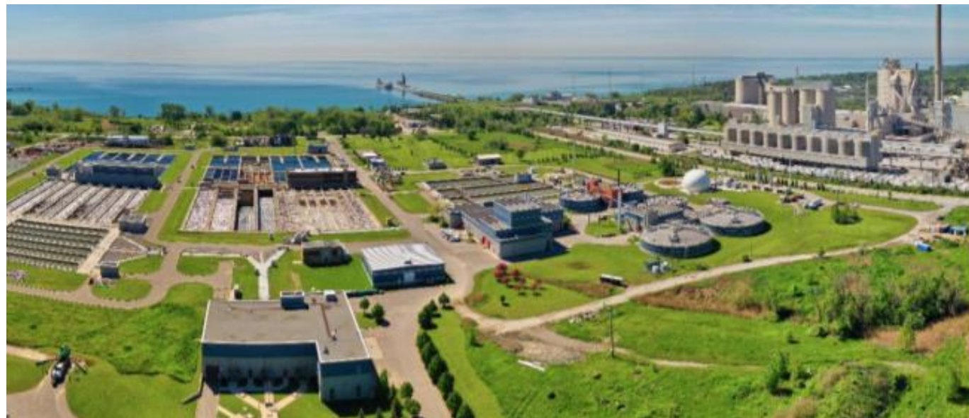
Clarkson Water Resource Recovery Facility (WRRF) (350 MLD)
