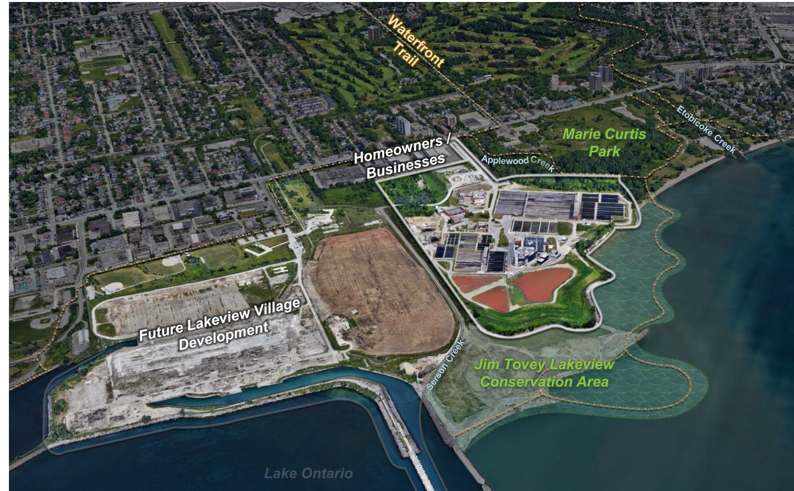
G.E. Booth Wastewater Treatment Plant
