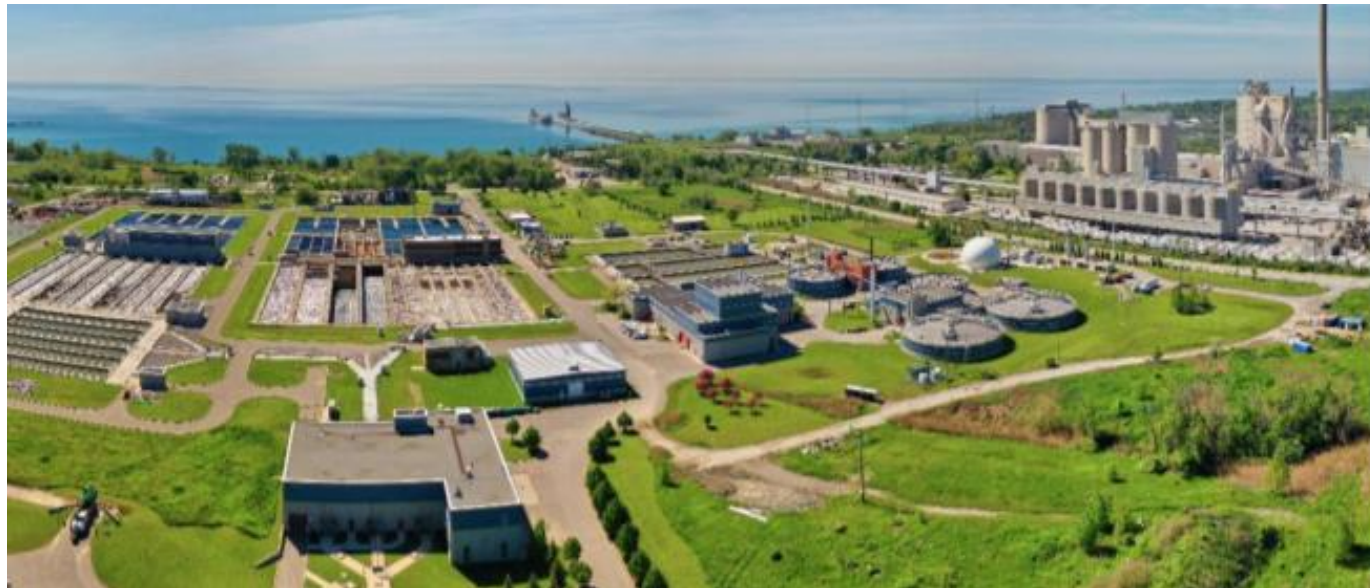
Clarkson Wastewater Treatment Plant (350 MLD)
