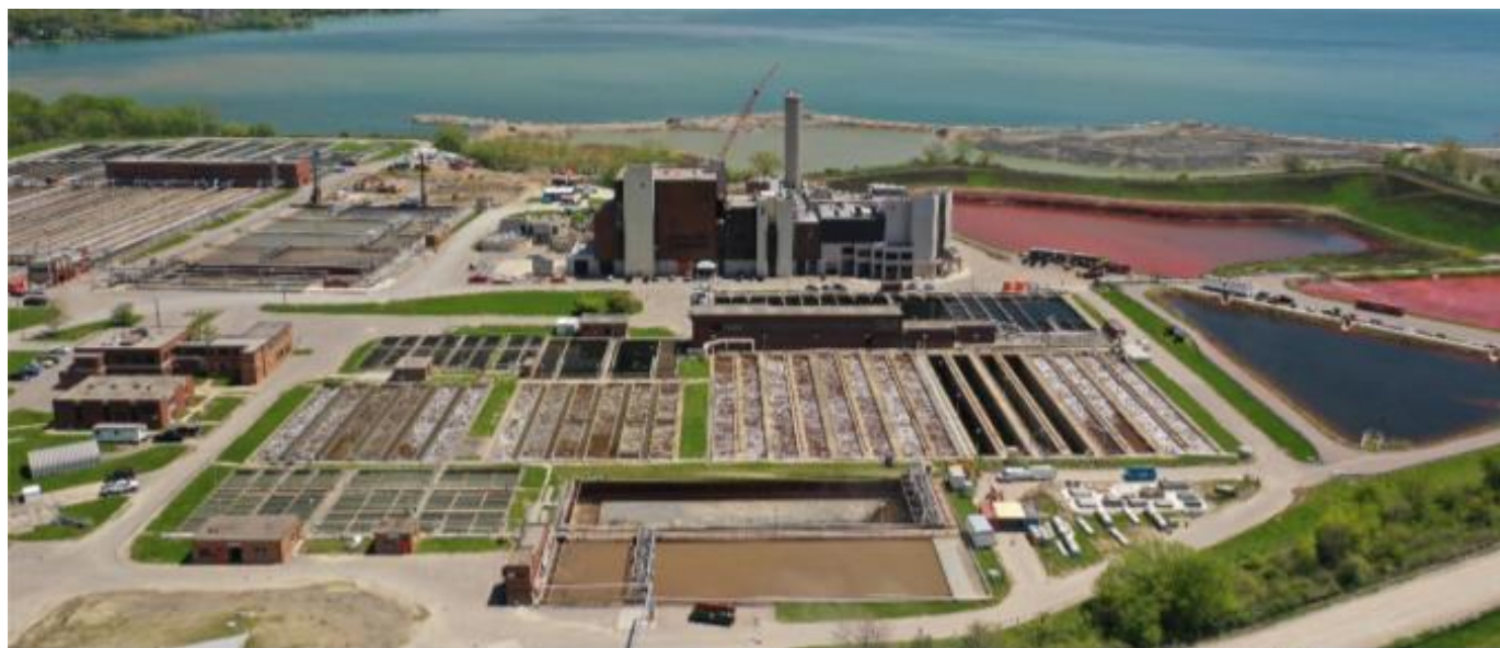
G.E. Booth Wastewater Treatment Plant
