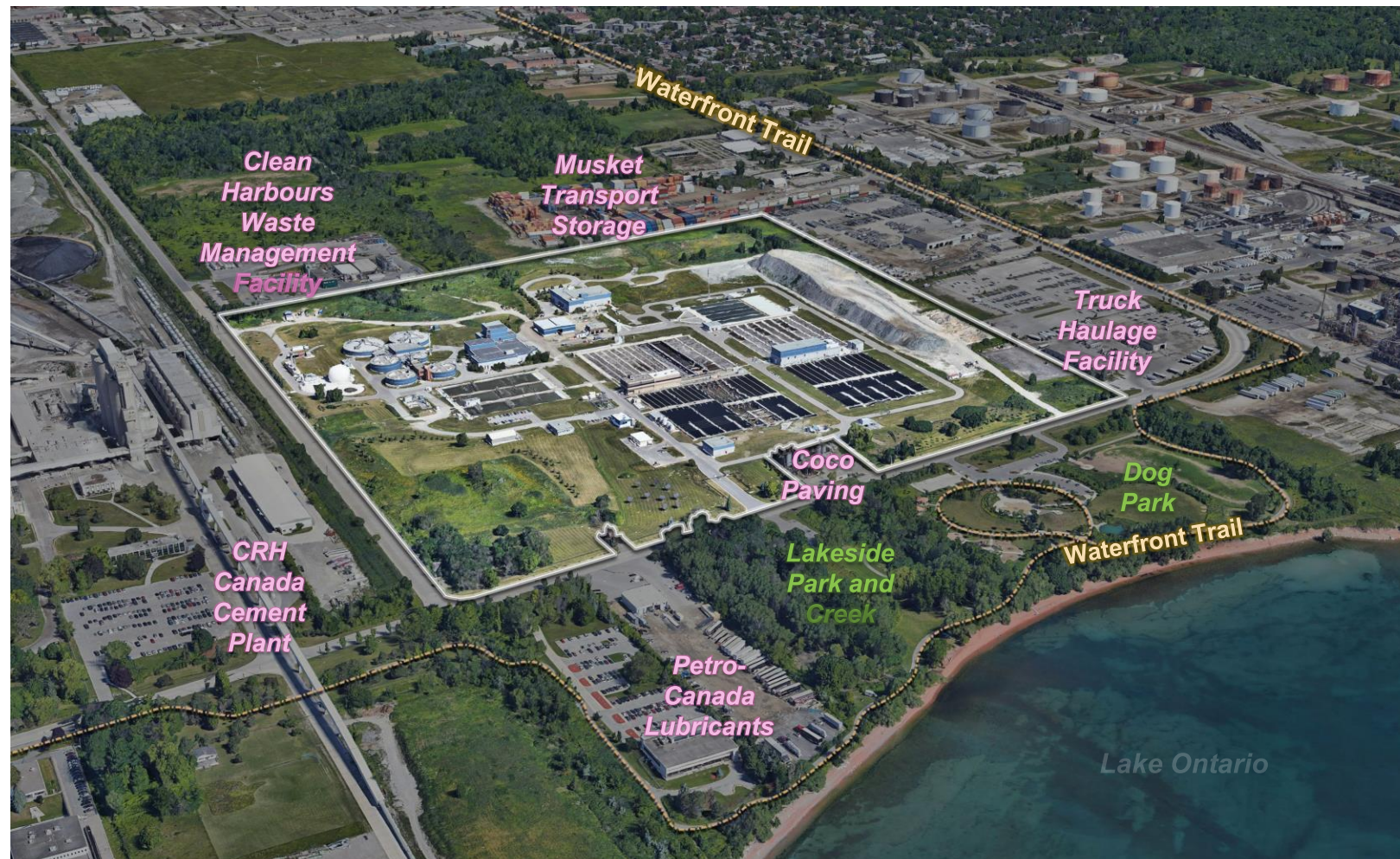
Clarkson Wastewater Treatment Plant
