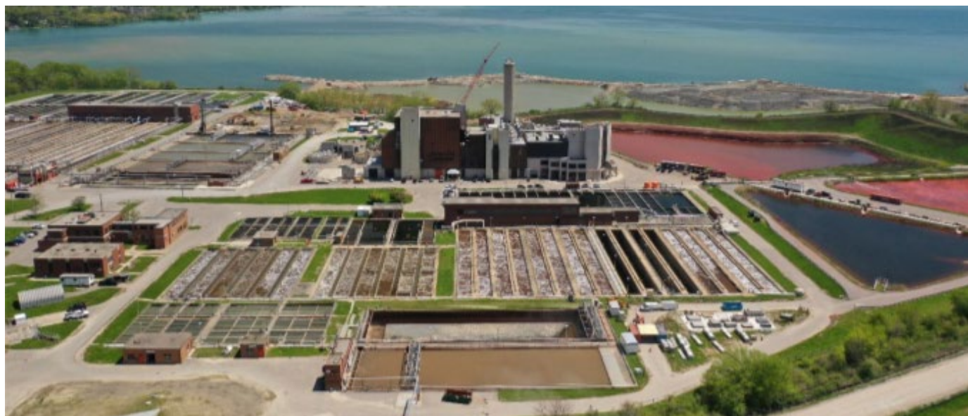
G.E. Booth Wastewater Treatment Plant
