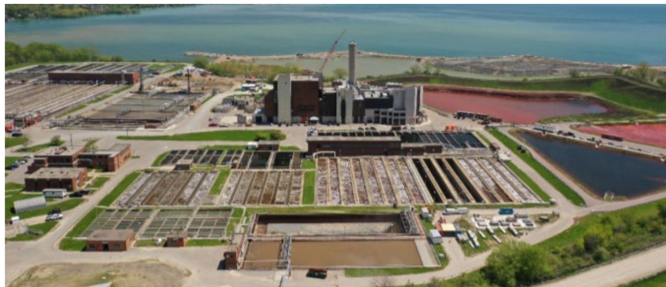
G.E. Booth Wastewater Treatment Plant
