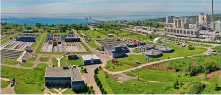
Clarkson Wastewater Treatment Plant
