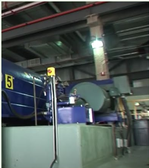
Thickening & Dewatering (G.E. Booth Wastewater Treatment Plant)
