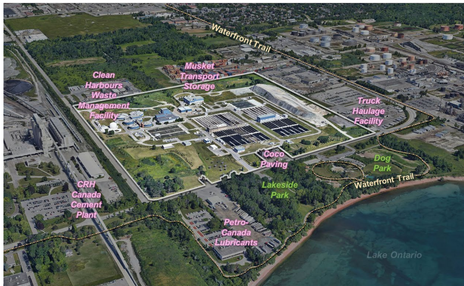
Clarkson Wastewater Treatment Plant
