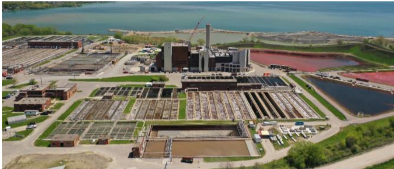
G.E. Booth Wastewater Treatment Plant (518 MLD)
