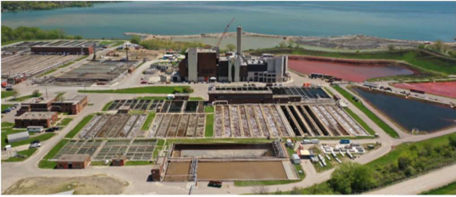
G.E. Booth Wastewater Treatment Plant
