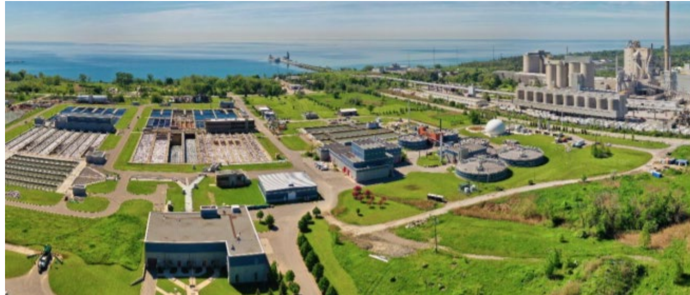
Clarkson Wastewater Treatment Plant
