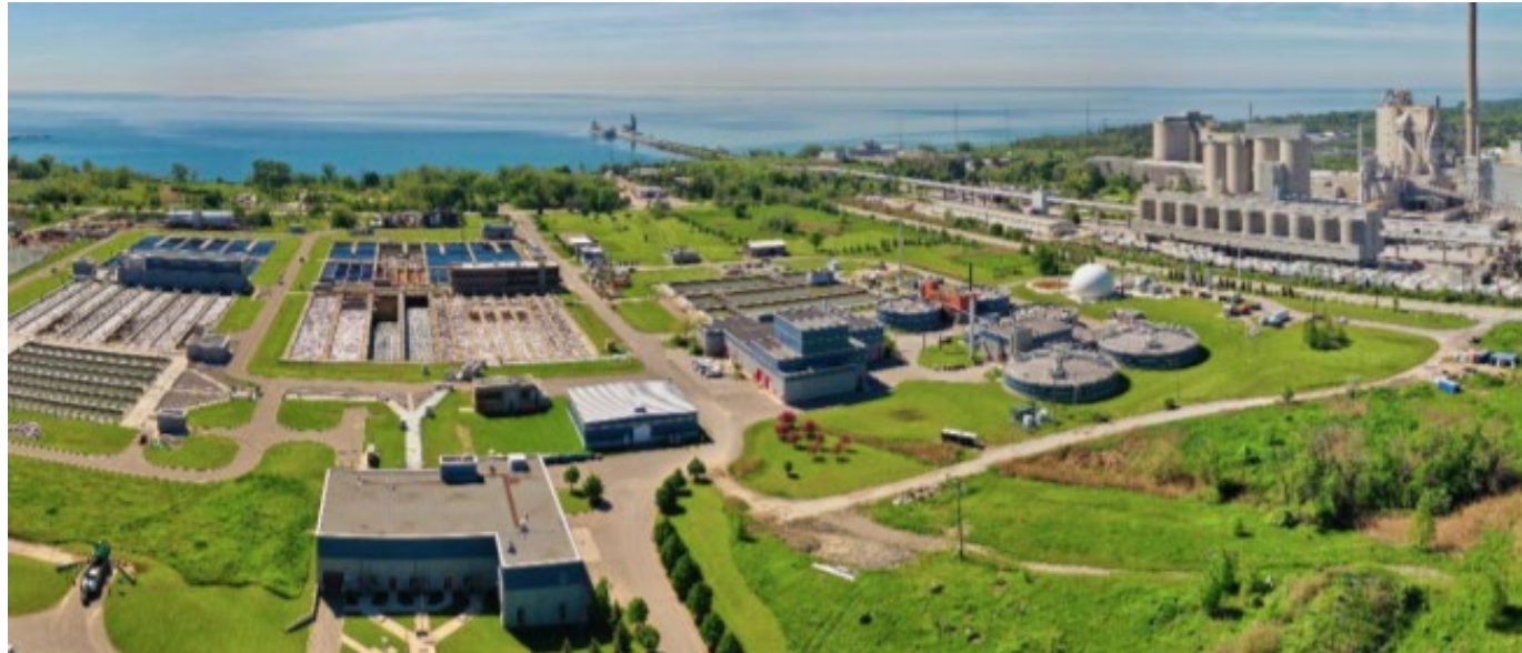
Clarkson Wastewater Treatment Plant
