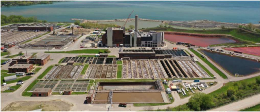
G.E. Booth Wastewater Treatment Plant
