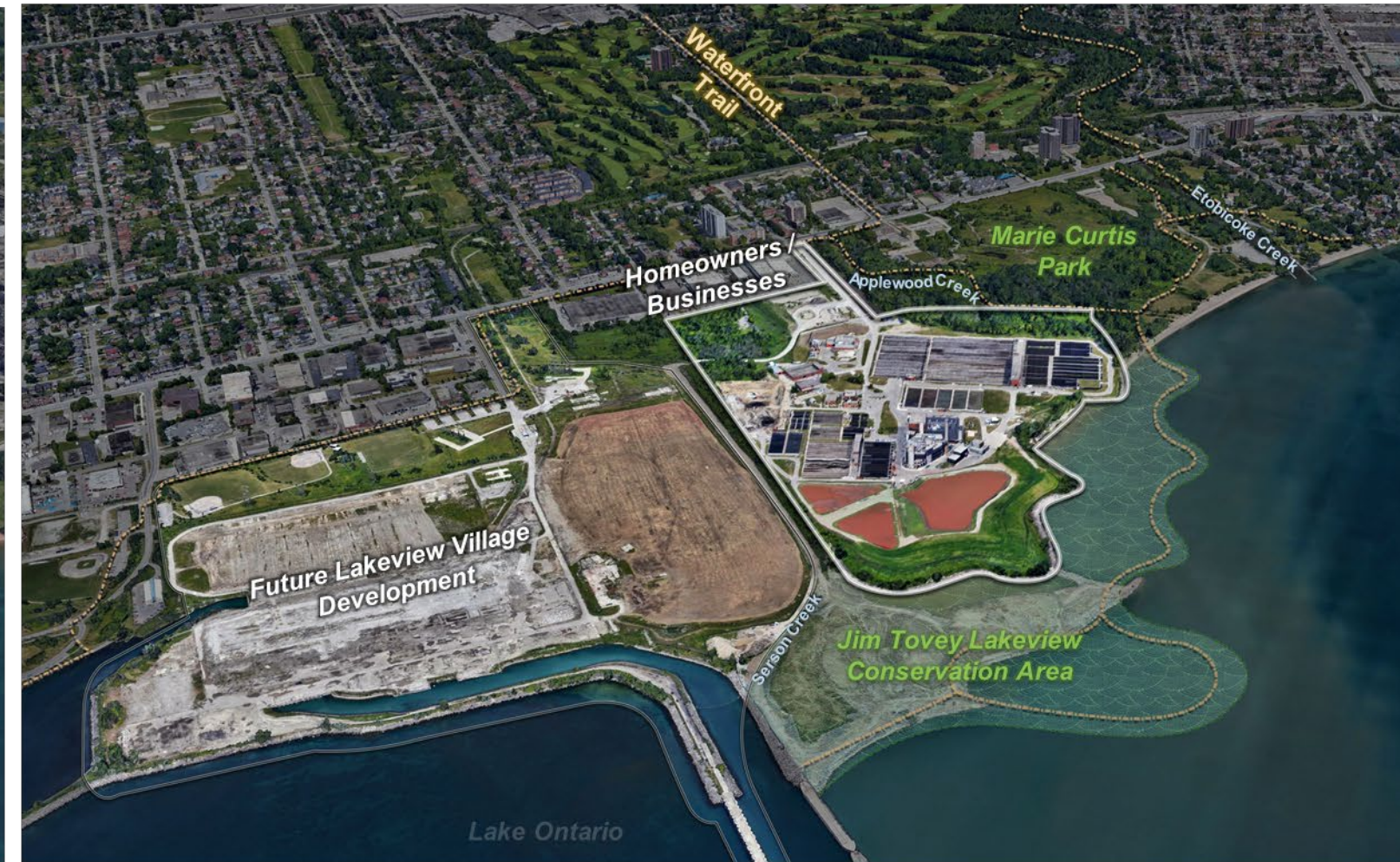
G.E. Booth Wastewater Treatment Plant
