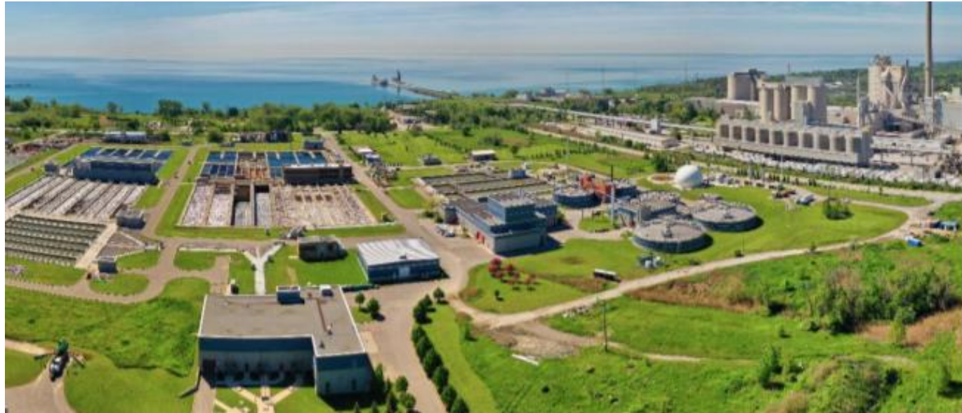
Clarkson Wastewater Treatment Plant (350 MLD)
