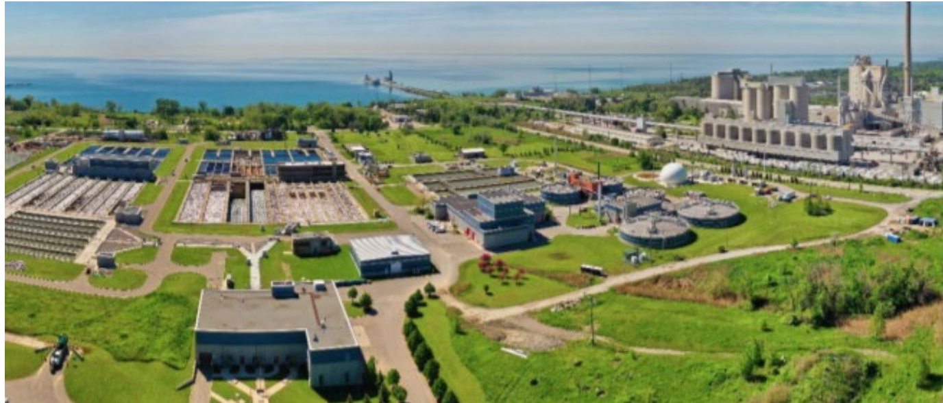
Clarkson Wastewater Treatment Plant
