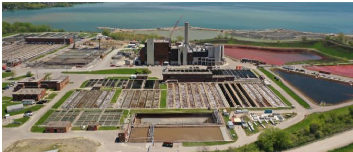
G.E. Booth Wastewater Treatment Plant (518 MLD)
