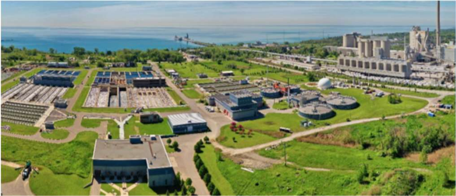
Clarkson Wastewater Treatment Plant
