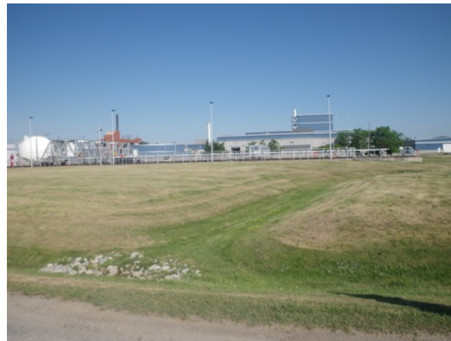
Image 20: View of graded landscape and existing structures near centre of Clarkson WWTP.
