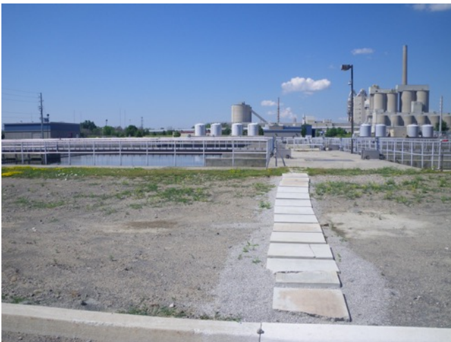
Image 7: View of extant structures and disturbed landscape at Clarkson WWTP.
