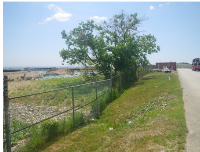
Image 24: View of extant paved road and artificial landscape at G.E. Booth WWTP, with ongoing Lake Ontario reclamation works visible.
