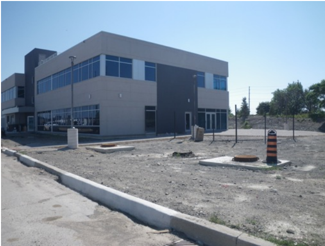
Image 5: View of recently constructed administration building.
