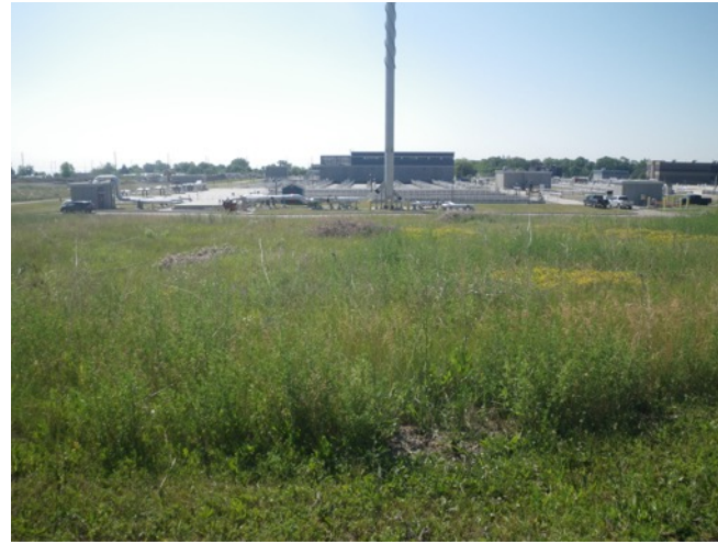
Image 22: View of extant paved surfaces and structures in the east of Clarkson WWTP.
