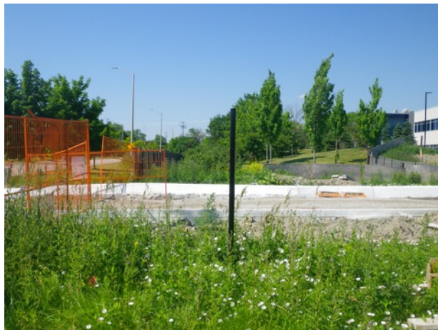
Image 4: View of access road under construction and flagged utility line (bottom left) near southeast corner of Clarkson WWTP.
