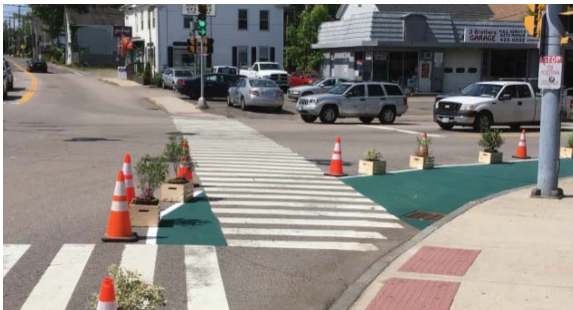
Exhibit 3-3: Example of a local street curb extension demonstration project, permitted by the transportation authority as a temporary condition
