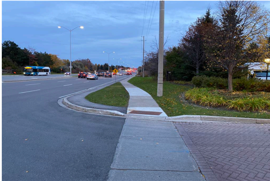
Image 49: LID area 8 showing slope, facing southeast
