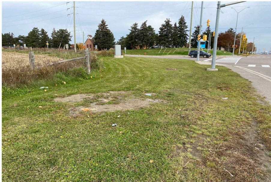
Image 15: LID area 5 showing disturbance along roadway, facing north
