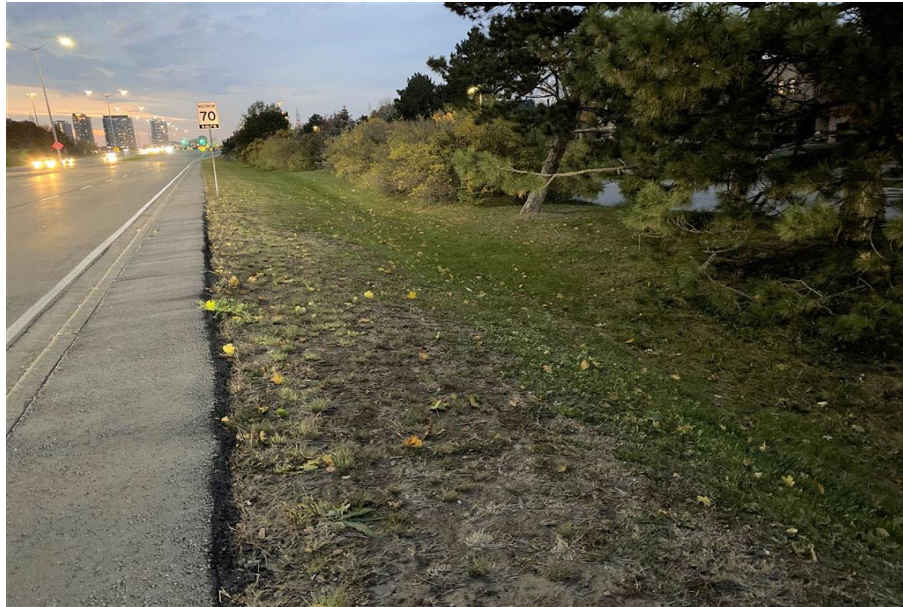
Image 47: LID area 8 showing slope, facing northwest
