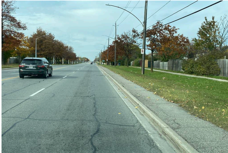
Image 57: LID area 9 showing paved disturbance, facing west
