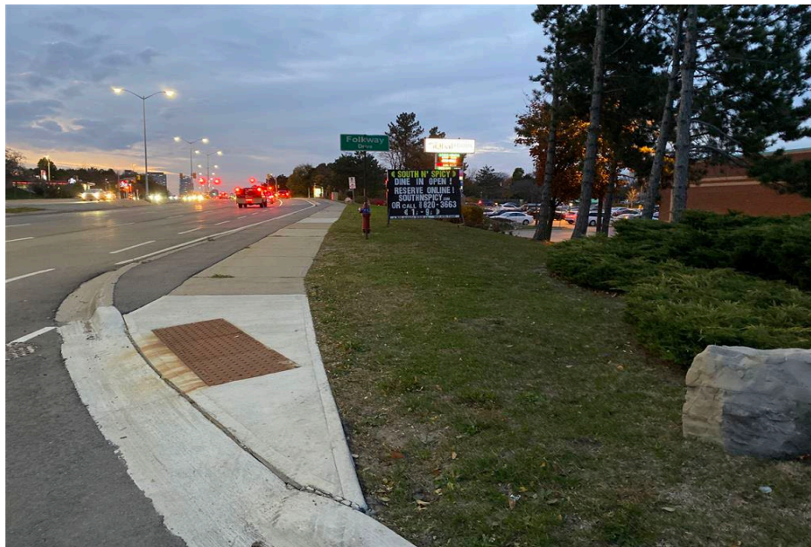
Image 48: LID area 8 showing slope, facing northwest
