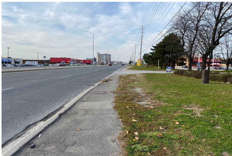
Image 38: LID area 7 showing disturbance, facing northwest
