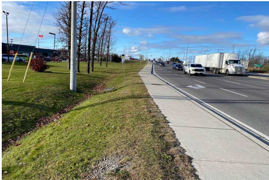
Image 41: LID area 7 showing slope, facing northwest
