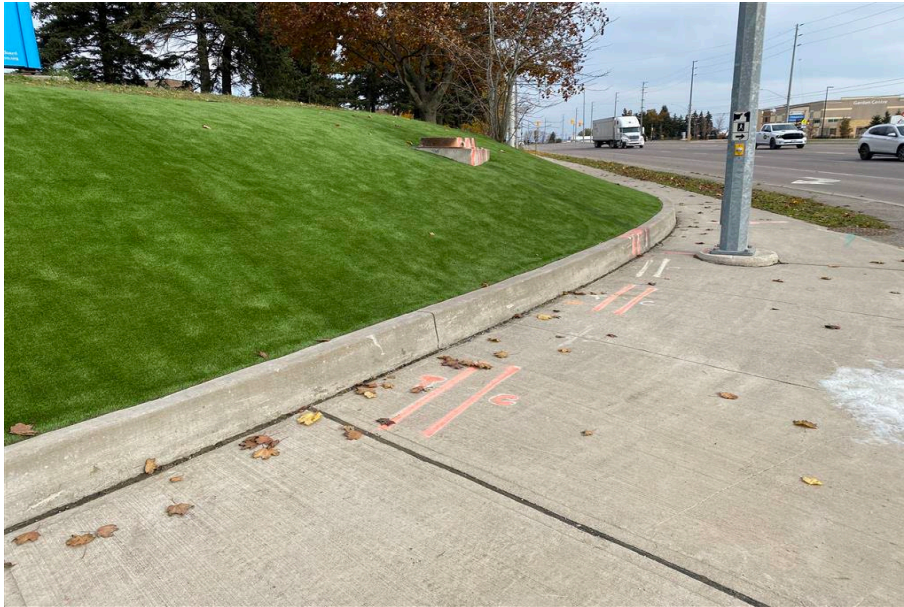
Image 17: LID area 5 showing slope and built up area, facing east
