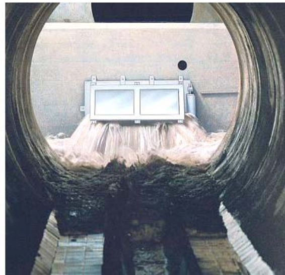
I&I STORAGE pipe with flushing
