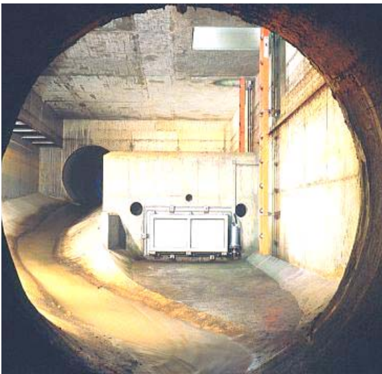
I&I STORAGE pipe with flushing
