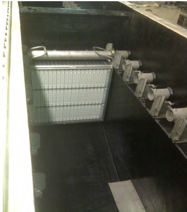
Figure 2: A membrane cassette containing 60 modules.
