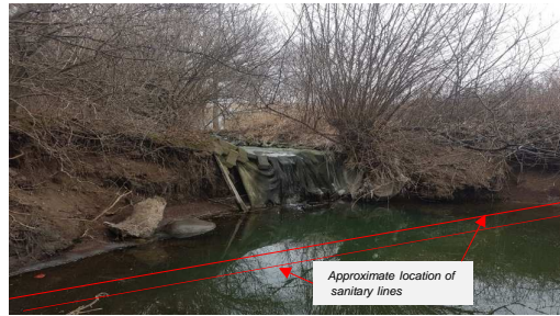
Peel Village Golf Course Sanitary Infrastructure Protection
