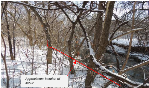
Derry Greenway Sanitary Infrastructure Protection
