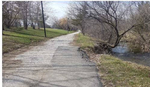
Brandon Gate Park Bank Stabilization and Infrastructure Protection
