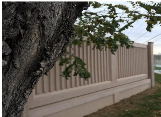
Finch Avenue - After Construction
