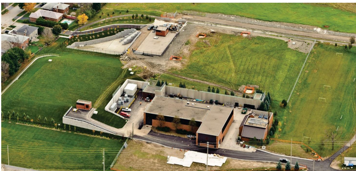
Figure 8. Herridge Reservoir and Pumping Station
