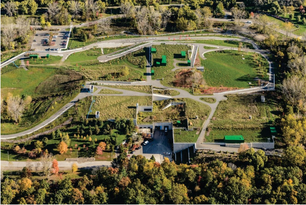
Figure 6. Lorne Park Water Treatment Plant
