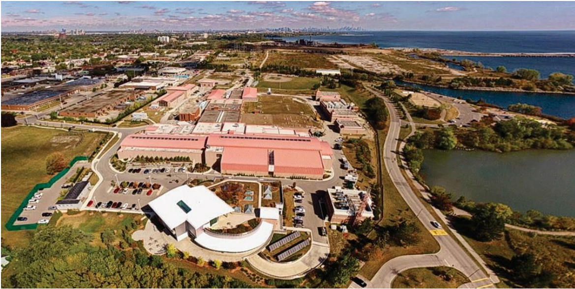
Figure 5. Arthur P. Kennedy Water Treatment Plant
