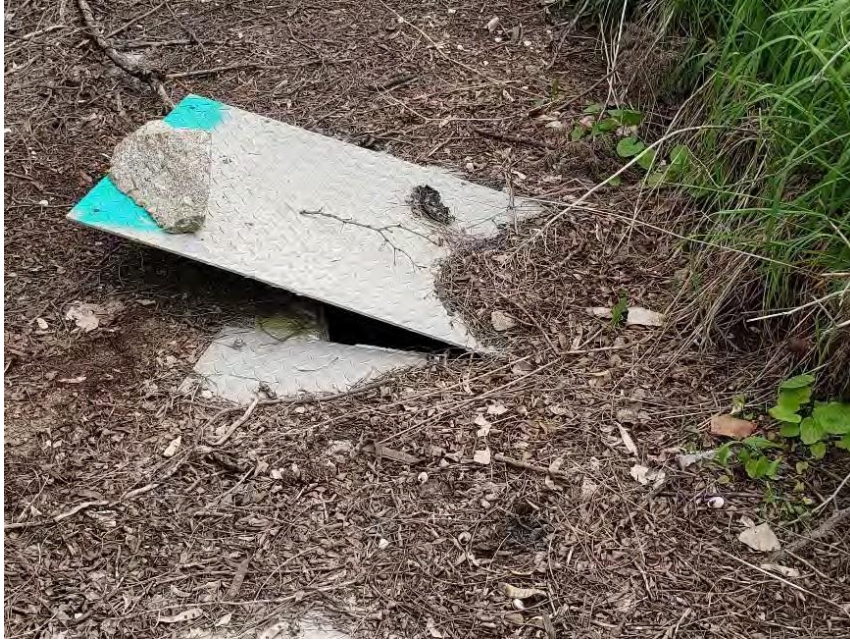
Figure 1-4. Removed Access Cover to Flume
