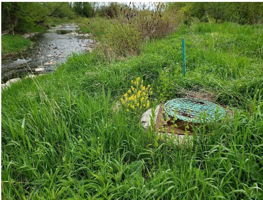
Figure 1-7. Maintenance Hole in Close Proximity to Etobicoke Creek
