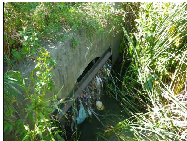
Tributary 1 of Mullet Creek: Outlet of pipe.
