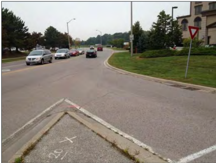
Photo 2-3: Receiving Leg for Northbound Traffic, North Side of Intersection
