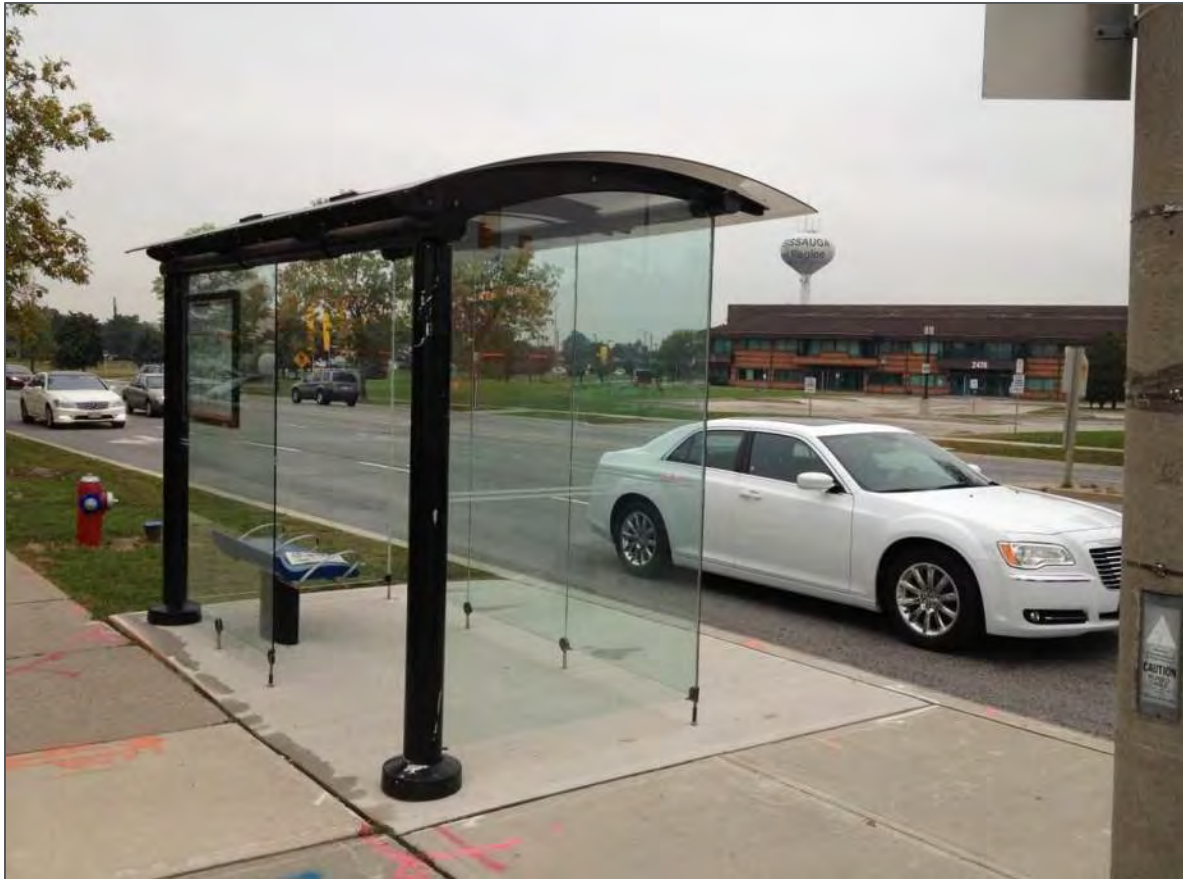
Photo 2-1: Transit Shelter at Southeast Corner of Intersection of Derry / Argentia
