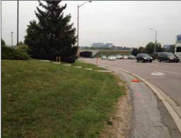
Photo 2-11: Splash Pad / Kill Strip on the North Side of Derry Road
