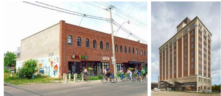
Above: Rendering of the Hines new Office buildings in the Junction. Below: Junction Breweries and Cafes & the MOCA Art Gallery / Office
