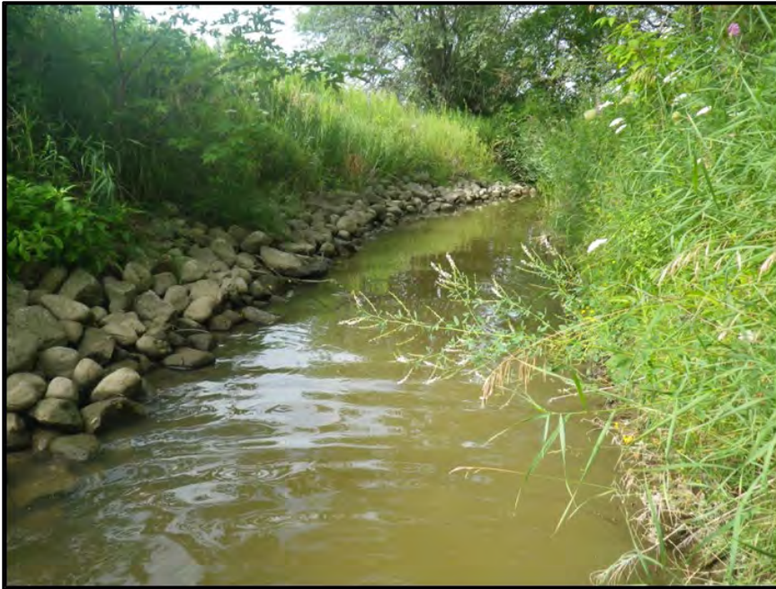
35. Reach C-8: riprap stone protection along Countryside Drive embankment and outside meander bend
