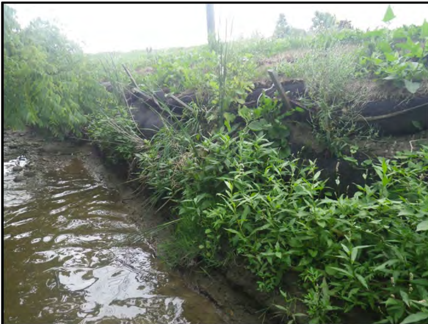
30. Reach C-7: vegetated coir-mat bank protection along south bank
