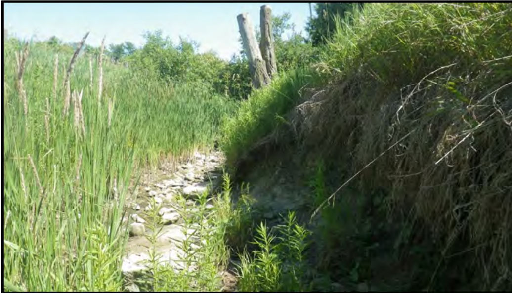
19. Reach C-5B: local erosion and undercutting of bank adjacent to road
