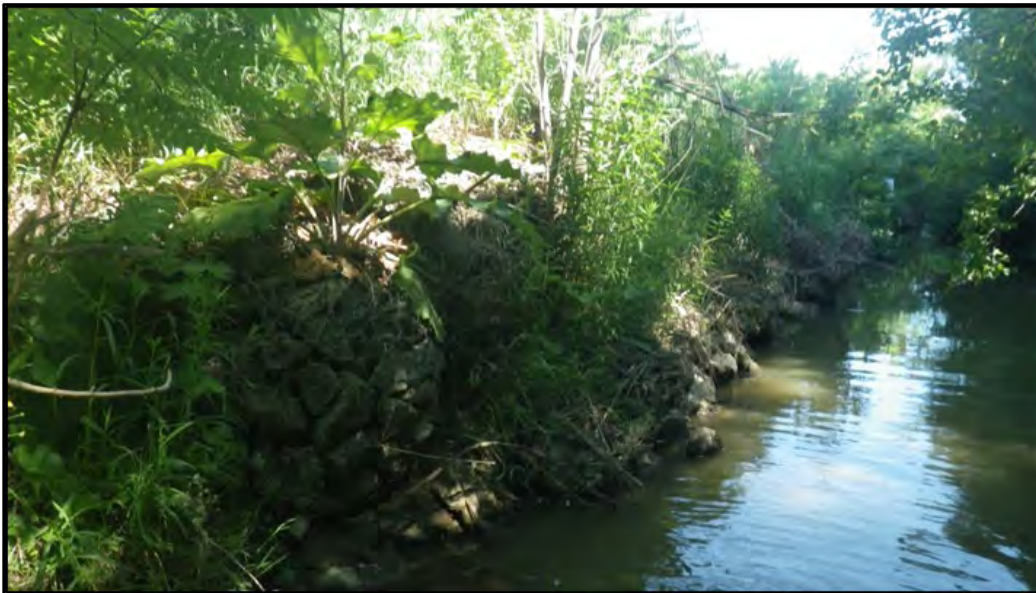
20. Reach C-5B: gabion baskets protect road embankment at the downstream extent of the reach; the gabion baskets are in poor condition with undercutting and failure of netting
