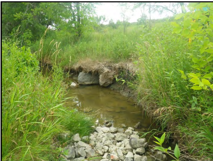
22. Reach C-6: boulder bank protection along outside meander bend; erosion and undercutting still occurring
