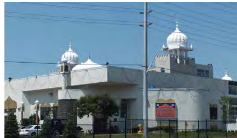
Ontario Khalsa Darbar (Sikh Temple) at Dixie Road north of Derry Road East, Brampton
