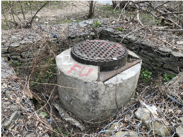
Plate 9: Detail of sewer located on the west bank of Etobicoke Creek.
