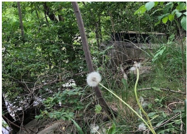
Photo 12: Maintenance hole to be decommissioned.
