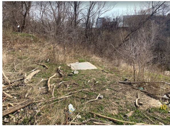
Photo 8: Embankment at drop structure area (April 6, 2021).
