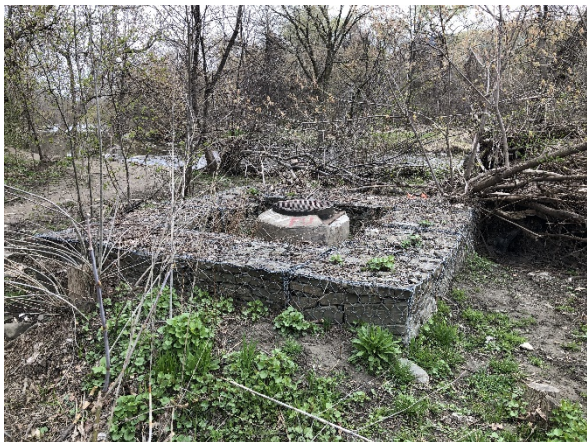
Plate 8: Sewer located on the west bank of Etobicoke Creek.
