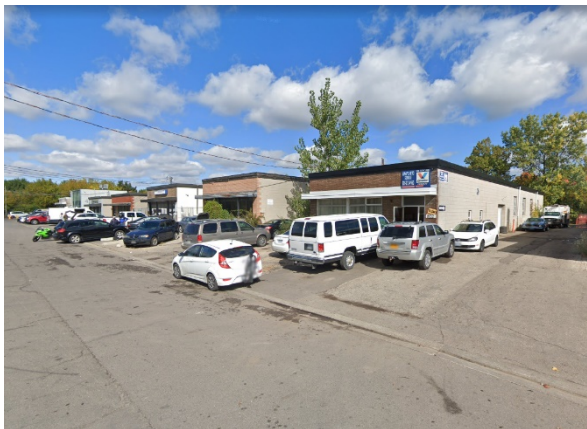
Plate 4: View along the northwest side of Mattawa Avenue (Google Streetview 2021).
