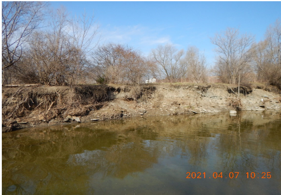
Cross Section 7 - Facing Right Bank
