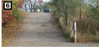
6 Grade Change at Abandoned EDC and Ex. Diversion Chamber. Potential impact access to construction site.
