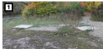
1 Ex. Junction Chamber – within proximity to adjacent watercourse and creek bank.
