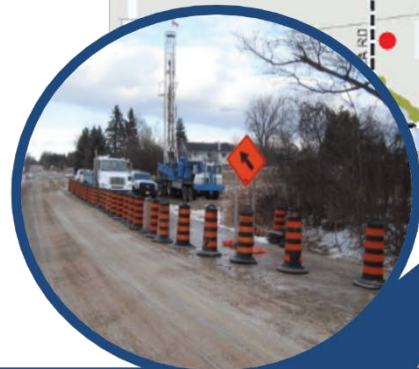
Site A Boston Mills Rd & Torbram Rd
