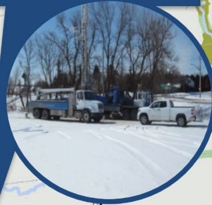
Site J Olde Baseline Rd at Dixie Rd
