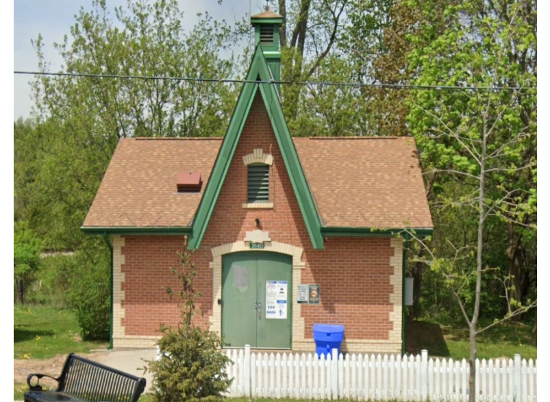
Alton Wells #3 & #4 Water Treatment Plant
