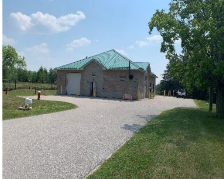
Palgrave Well #4 Water Treatment Plant
