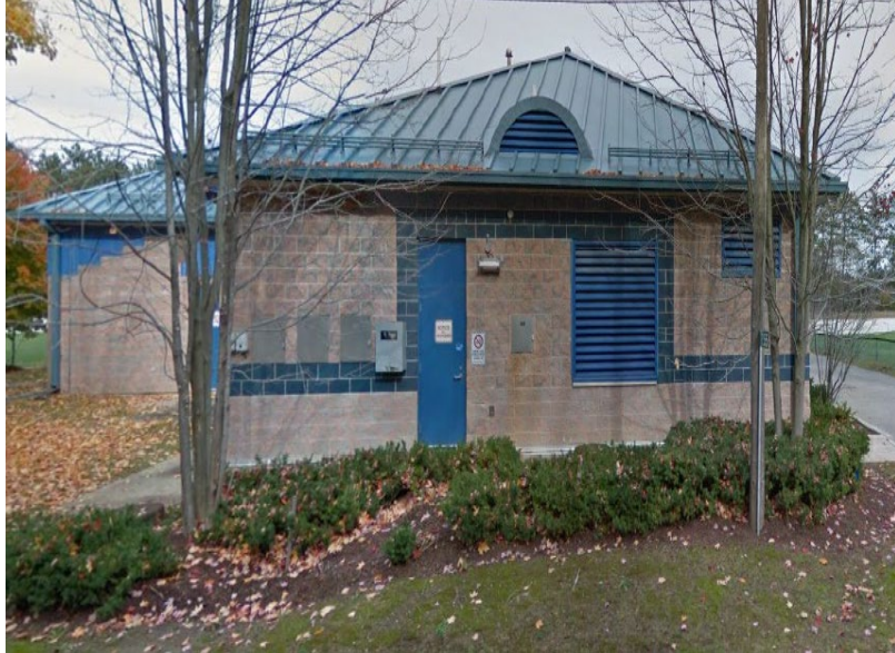
Palgrave Wells #2 & #3 Water Treatment Plant
