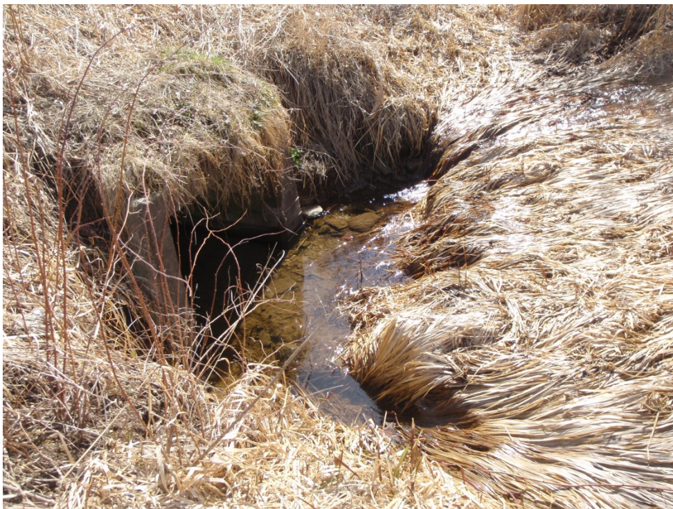
Photograph 6. Upstream end of Bovaird Drive culvert at watercourse 3a. March 30, 2010.
