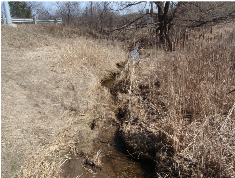
Photograph 8. Watercourse 3a downstream from Bovaird Drive culvert. March 30, 2010.
