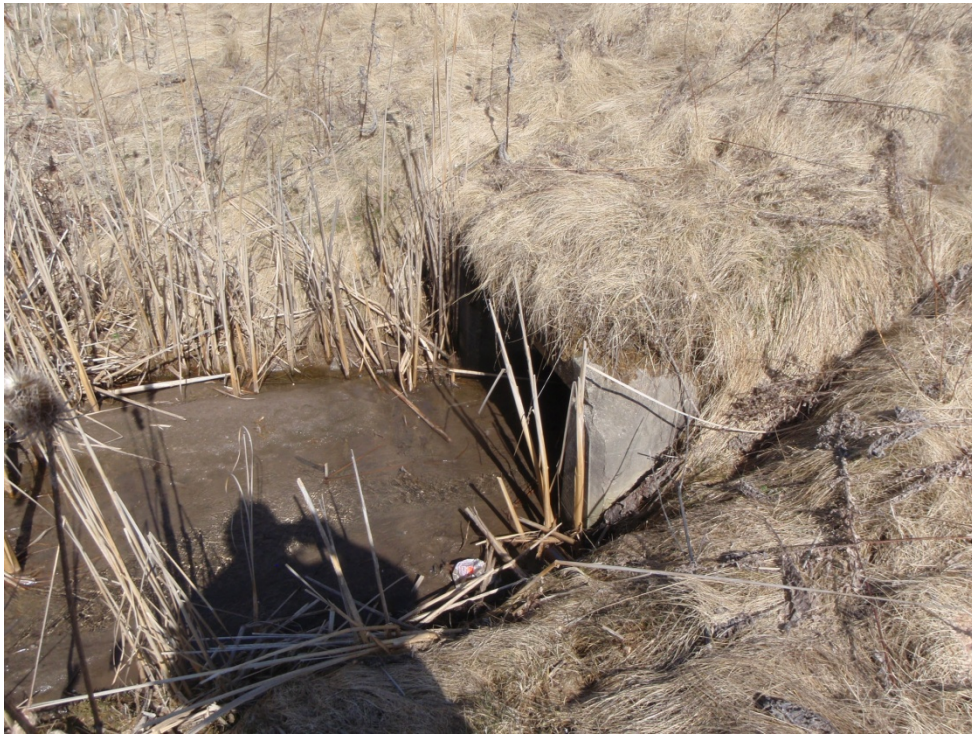
Photograph 4. Upstream end of Bovaird Drive culvert at watercourse 2b. March 30, 2010.
