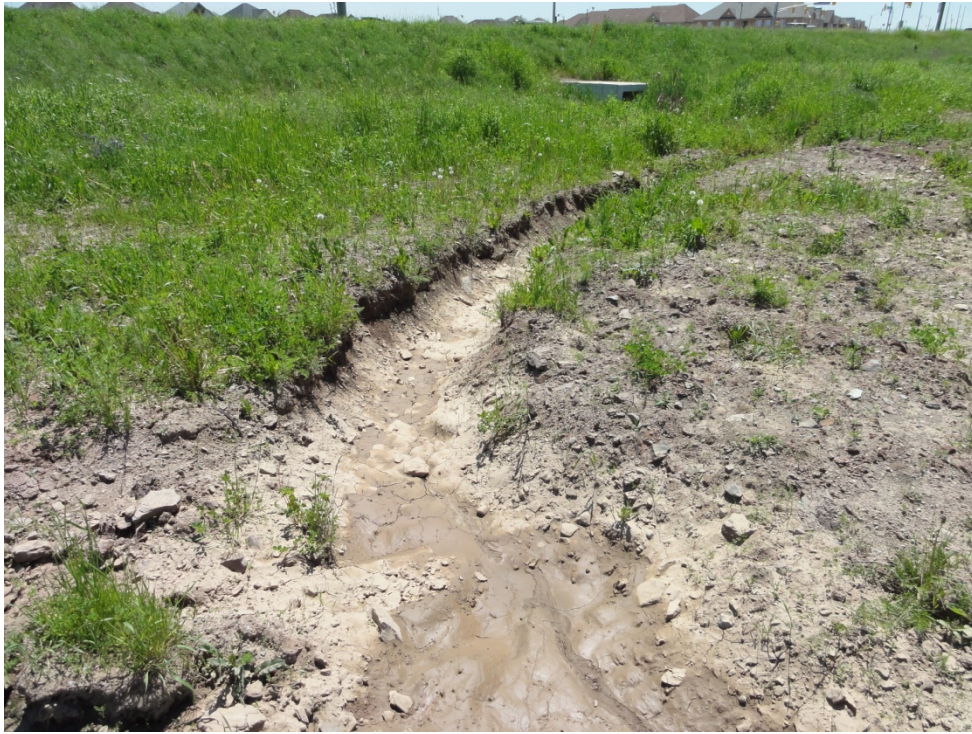
Photograph 17. Drainage feature in Fletcher's Creek watershed upstream from Bovaird Drive. June 6, 2011.
