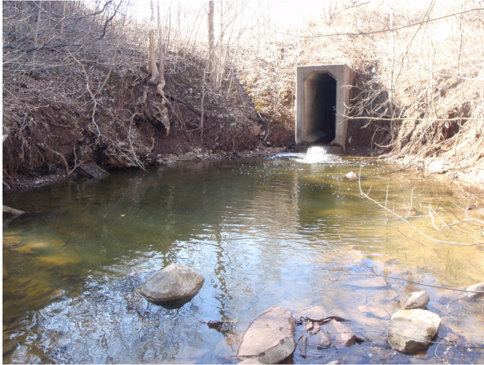
Photograph 1. Downstream end of culvert at watercourse 2a. March 30, 2010.
