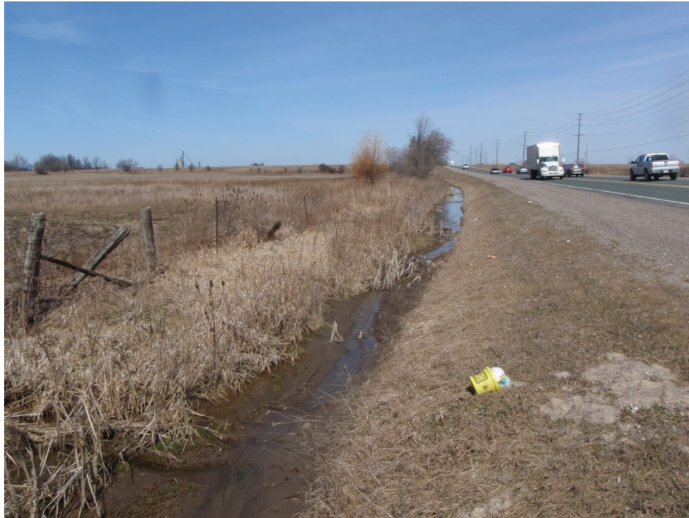
Photograph 10. Ditch flowing westerly to watercourse 3b on upstream side of Bovaird Drive. March 30, 2010.
