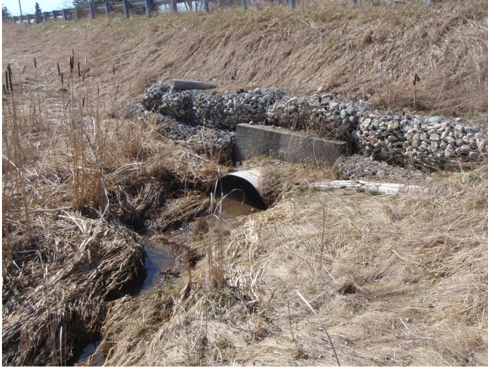
Photograph 7. Downstream end of Bovaird Drive culvert at watercourse 3a. March 30, 2010.
