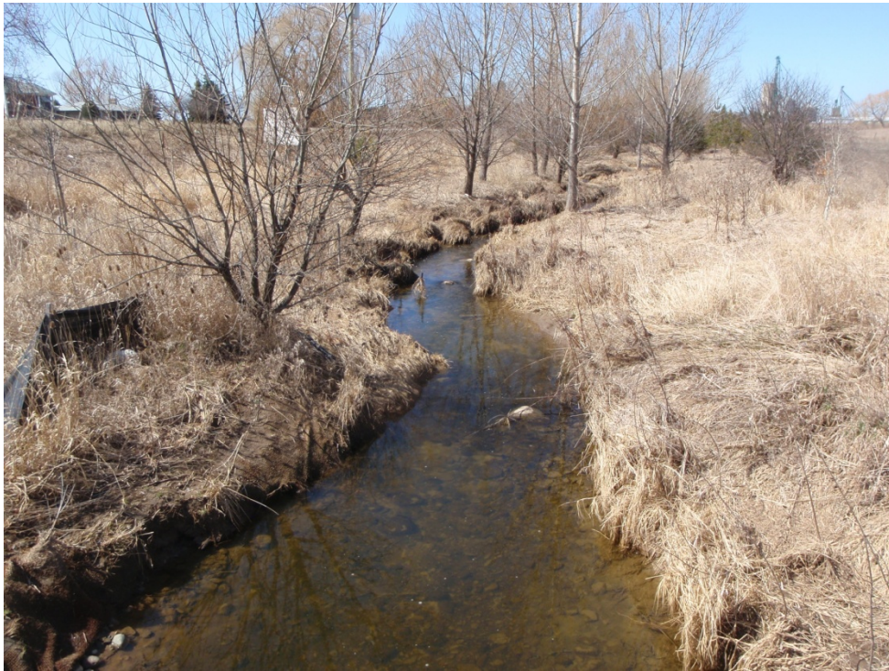
Photograph 14. Huttonville Creek looking upstream from Bovaird Drive culvert. March 30, 2010.
