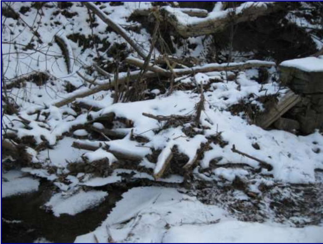
Photo 55 –Structure No. 14: Approximate Area of Inlet
