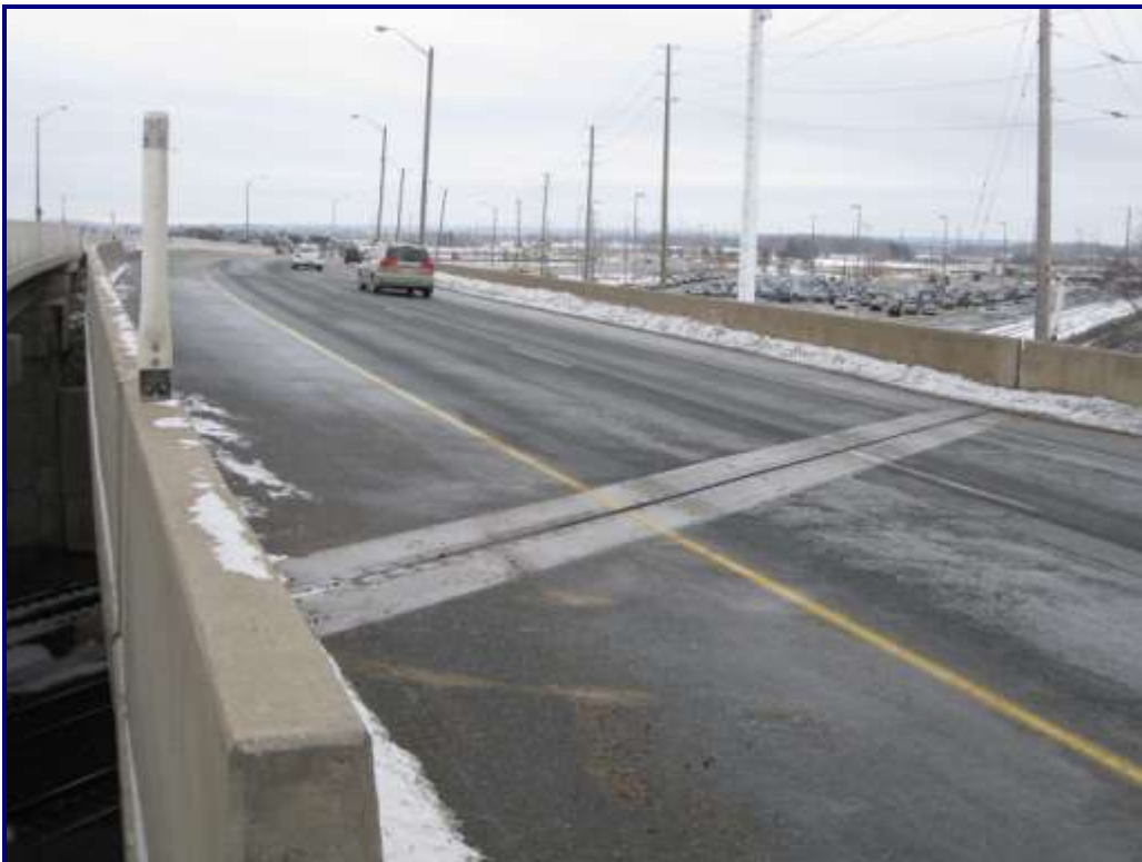
Photo 5 – Structure No. 2: West Bound Lanes
