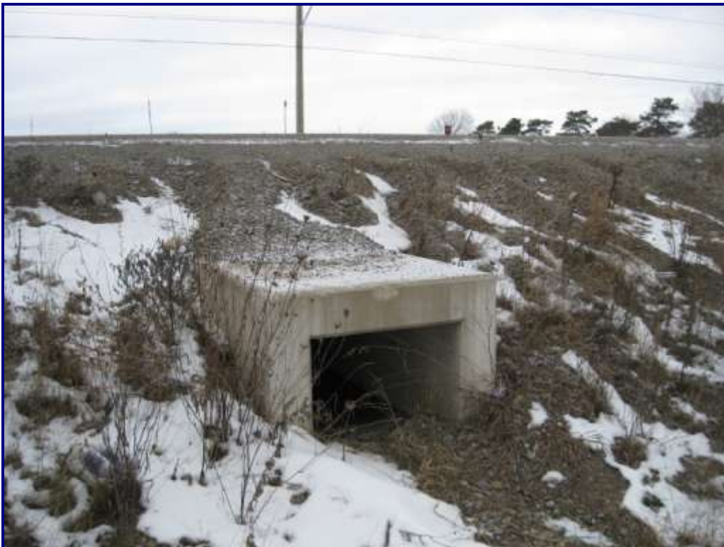
Photo 22 – Structure No. 4: South End of Culvert
