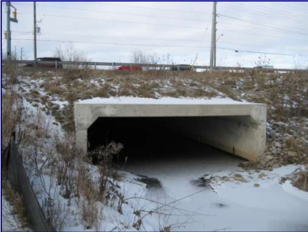
Photo 26 – Structure No. 5: South End of Culvert
