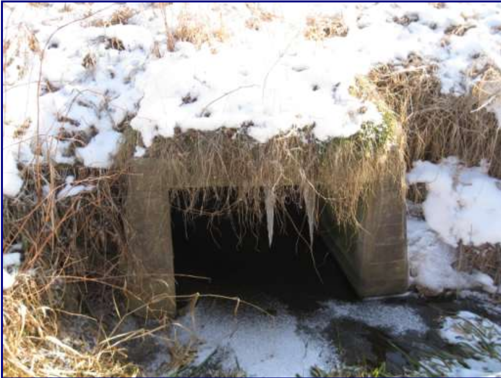
Photo 43 – Structure No. 11: North End of Culvert
