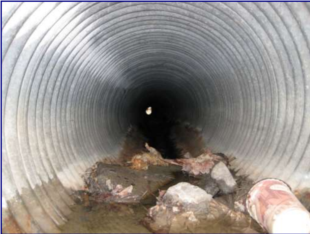
Photo 32 – Structure No. 8: West Barrel Looking East
