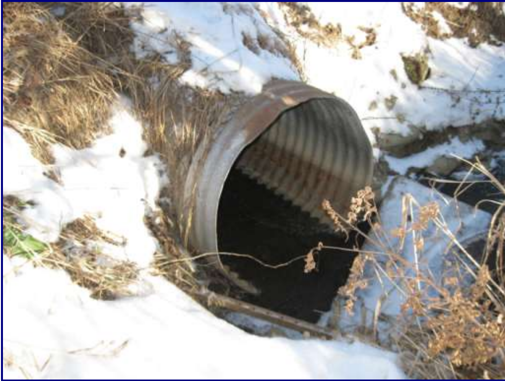
Photo 48 – Structure No. 12: West End of Culvert
