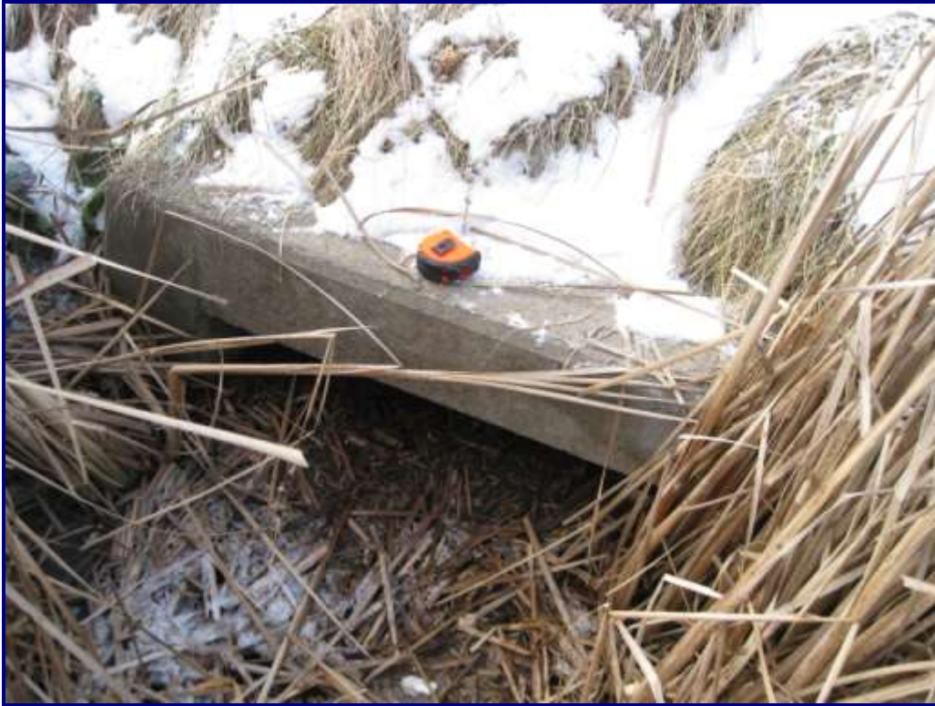
Photo 54 –Structure No. 13: South End of Culvert
