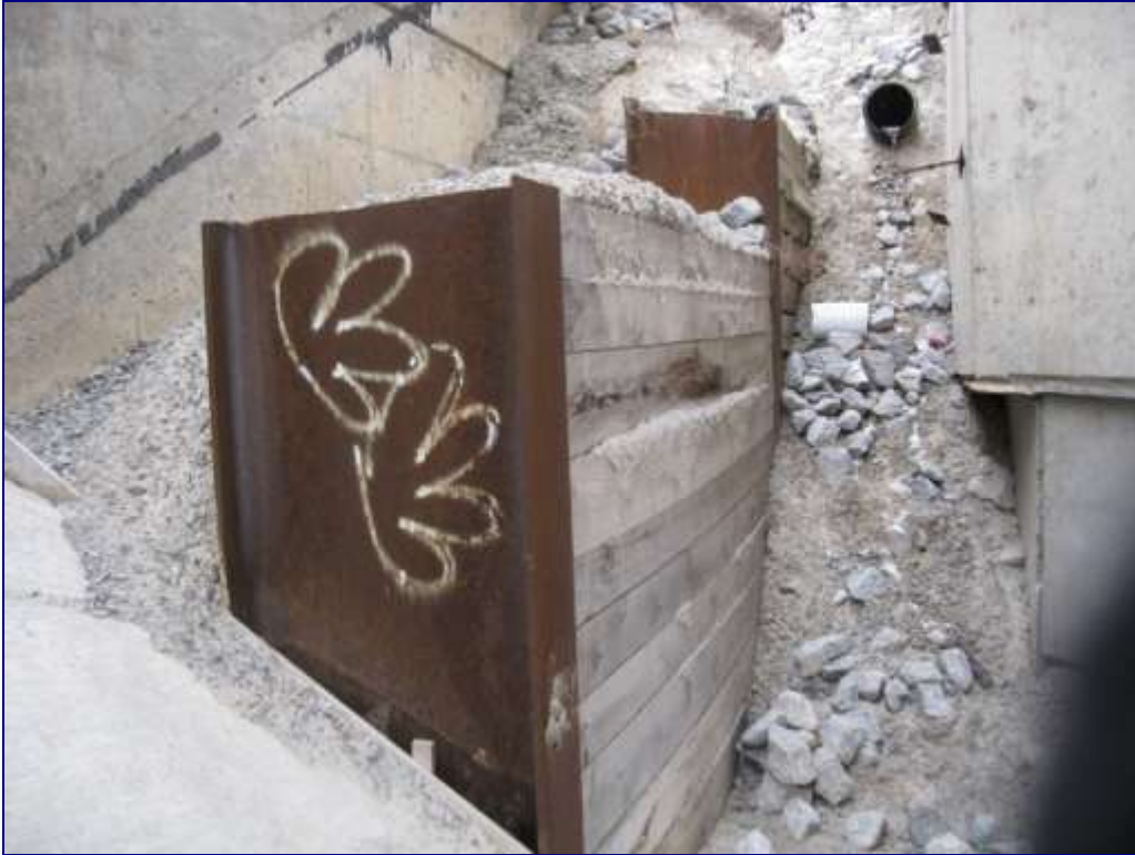
Photo 16 – Structure No. 2: Protection System Left in Place
