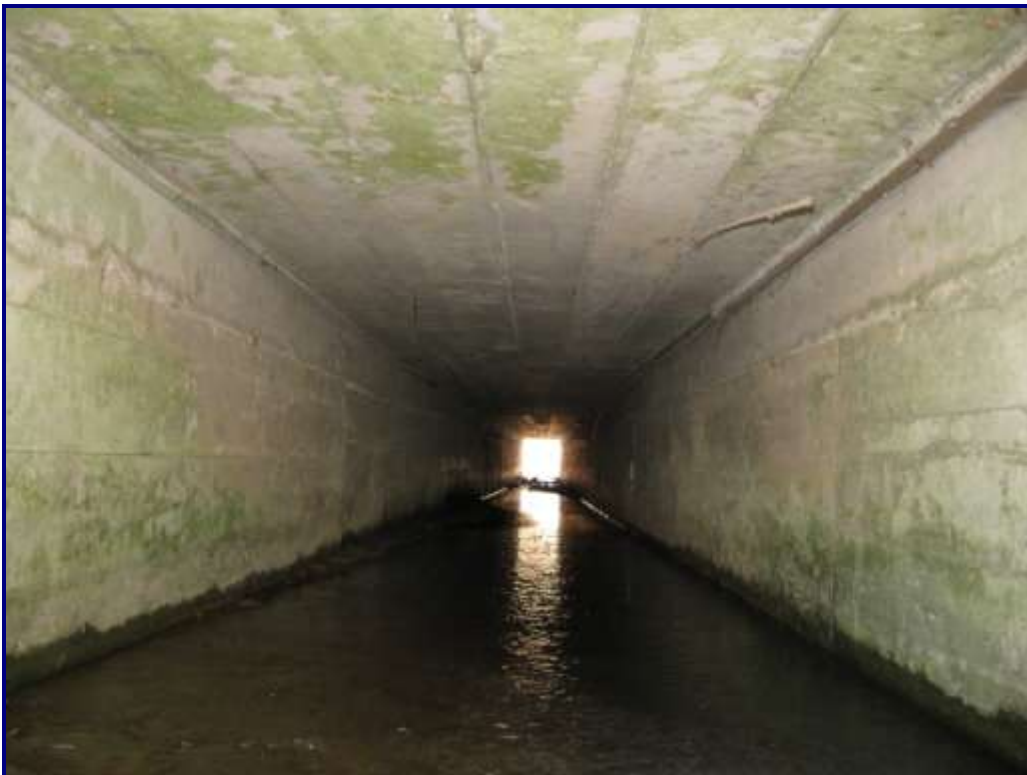
Photo 38 – Structure No. 9: South Barrel Looking North
