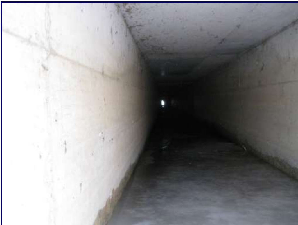
Photo 18 – Structure No. 3: North Barrel Looking South
