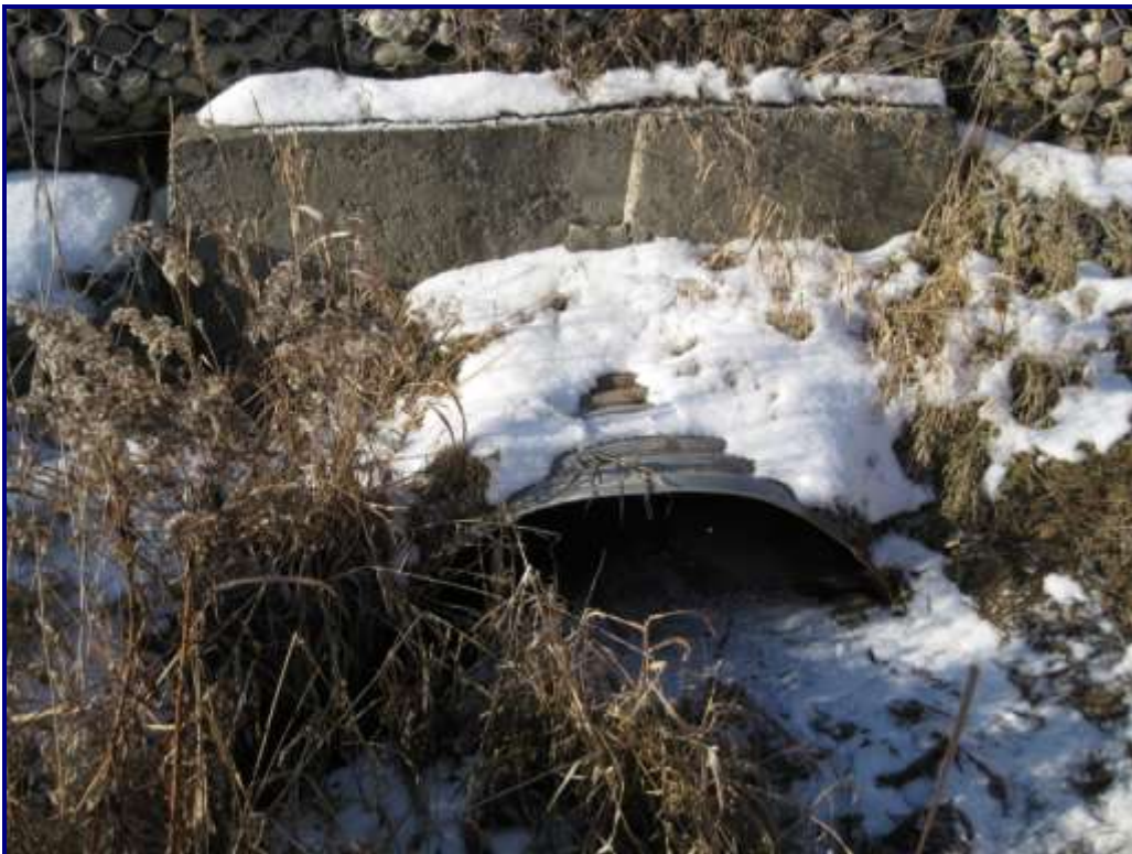
Photo 46 – Structure No. 11: South End of Culvert
