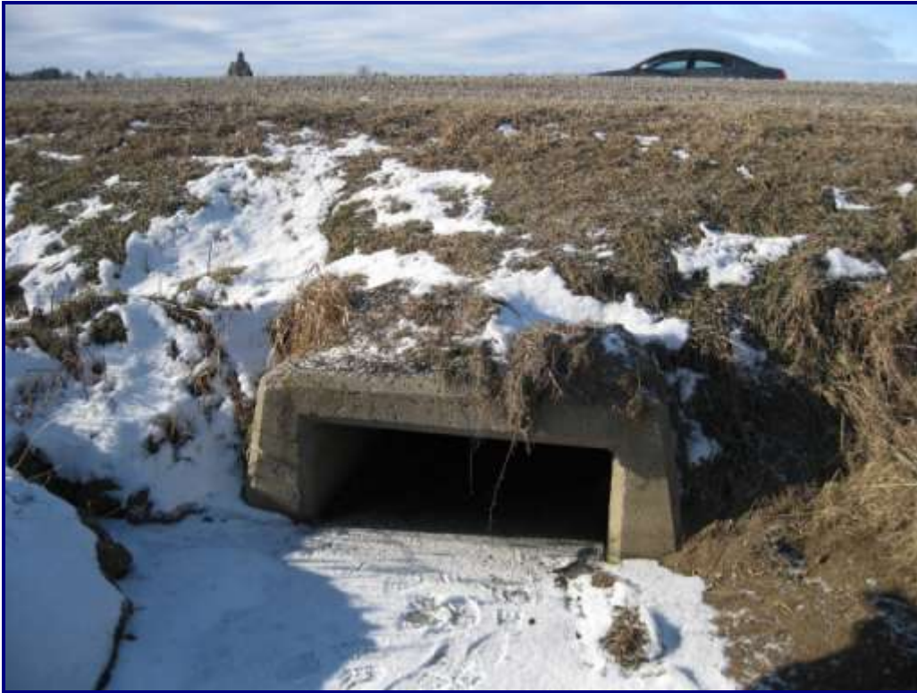
Photo 41 – Structure No. 10: South End of Culvert
