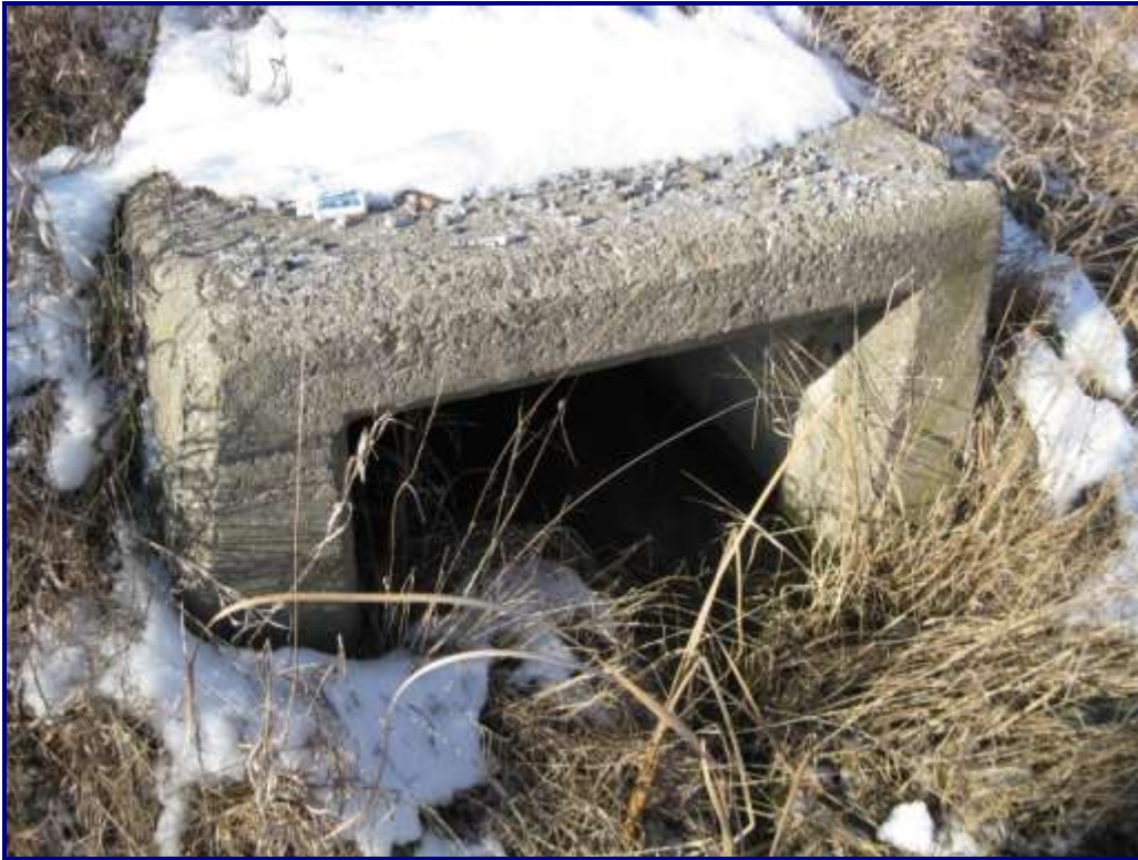
Photo 37 – Structure No. 9: South End of Culvert
