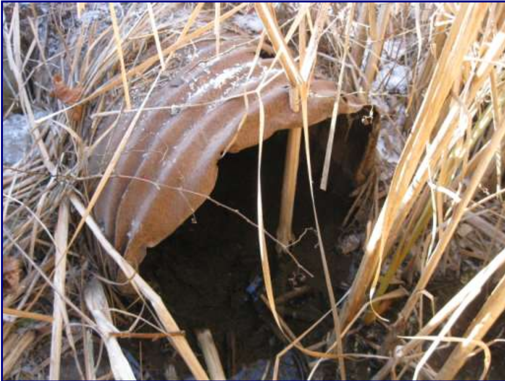
Photo 33 – Structure No. 8: East End of Culvert
