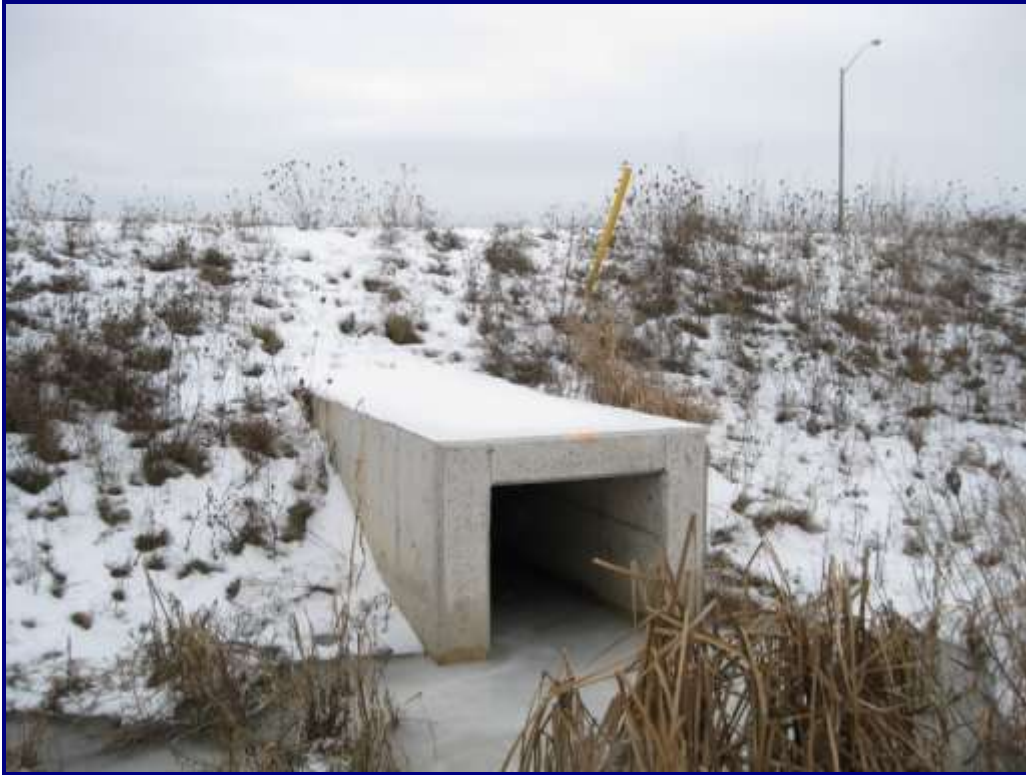
Photo 17 – Structure No. 3: North End of Structure
