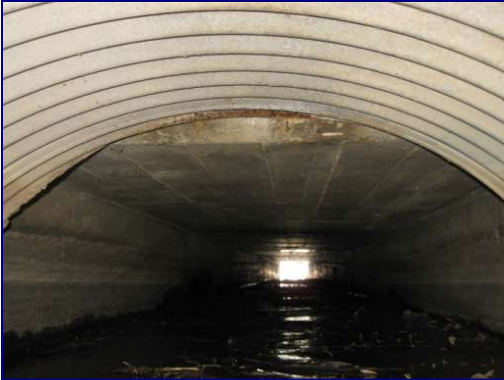
Photo 47 – Structure No. 11: South Barrel Looking North
