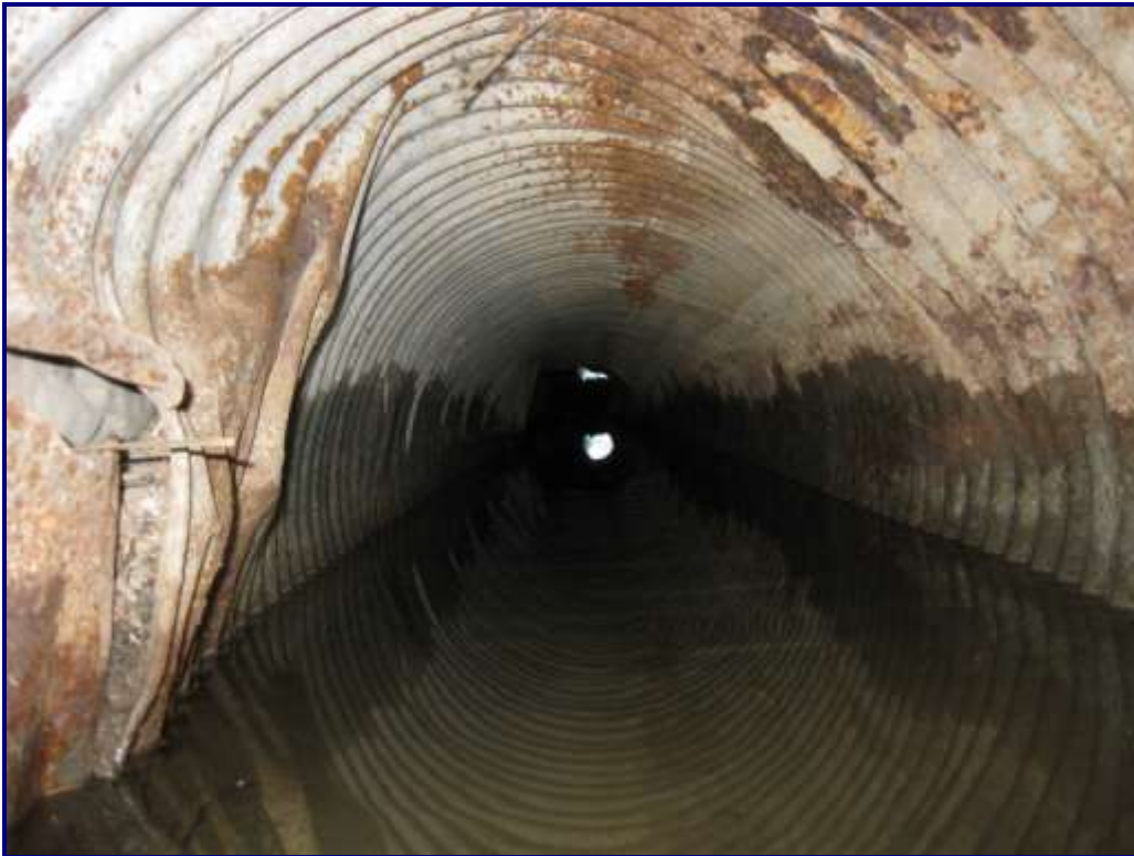
Photo 34 – Structure No. 8: East Barrel Looking West
