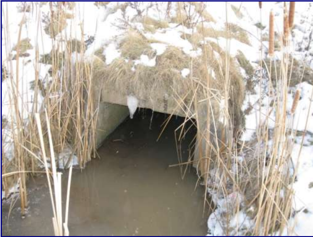
Photo 52 – Structure No. 13: North End of Culvert
