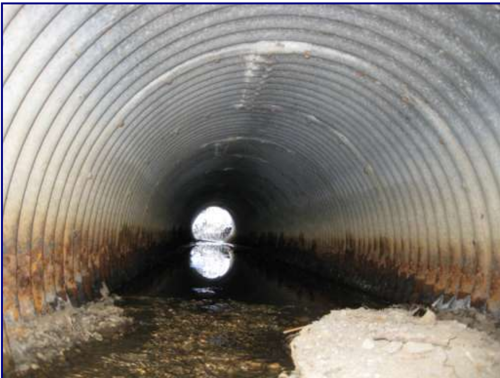
Photo 51 – Structure No. 12: East Barrel Looking West
