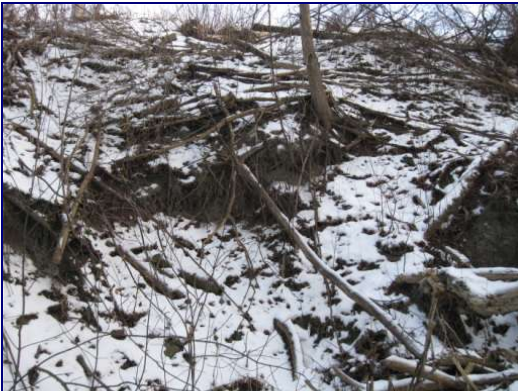
Photo 56 – Structure No. 14: North Slope Failure
