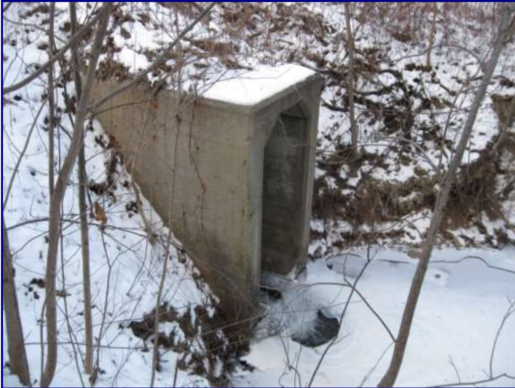
Photo 57 – Structure No. 14: South Culvert Outlet
