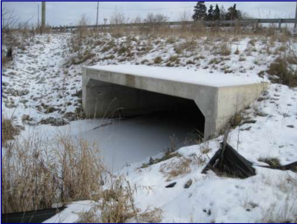
Photo 24 – Structure No. 5: North End of Culvert
