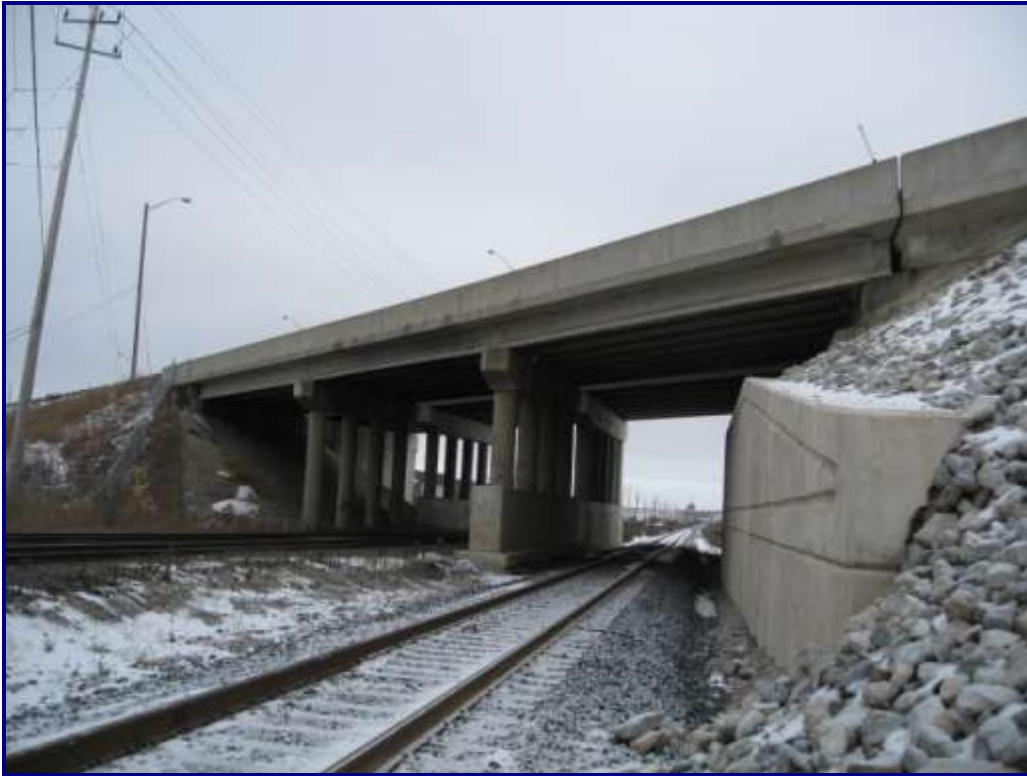
Photo 4 – Structure No. 2: North Elevation
