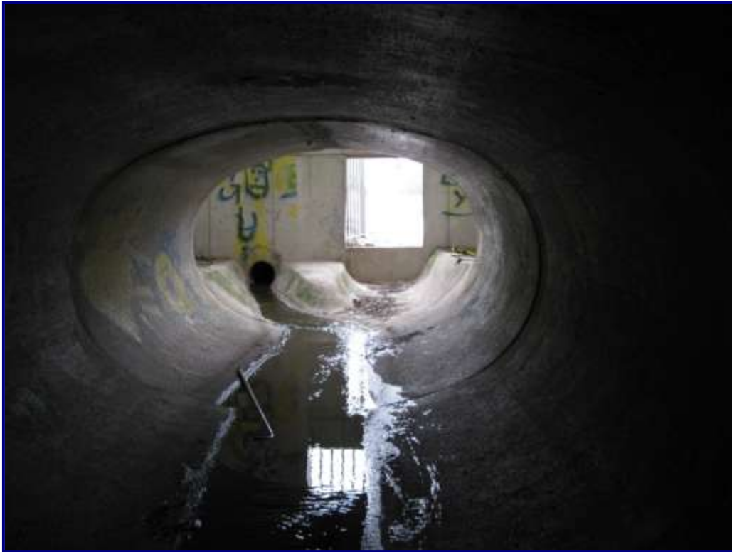
Photo 3 – Structure No. 1: Culvert Looking Upstream to Inlet Structure
