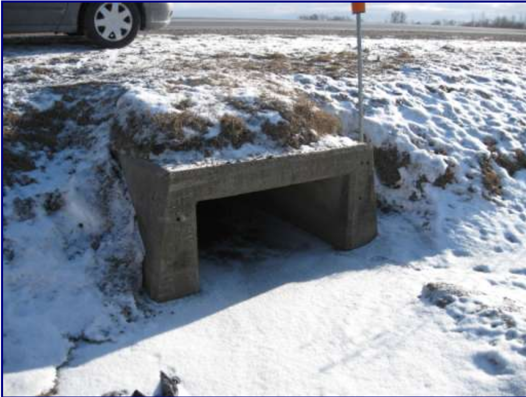
Photo 39 –Structure No. 10: North End of Culvert
