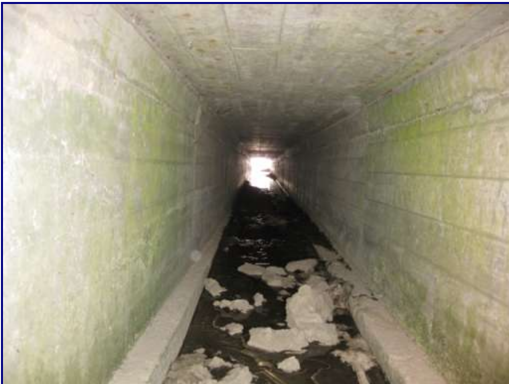
Photo 36 – Structure No. 9: North Barrel Looking South
