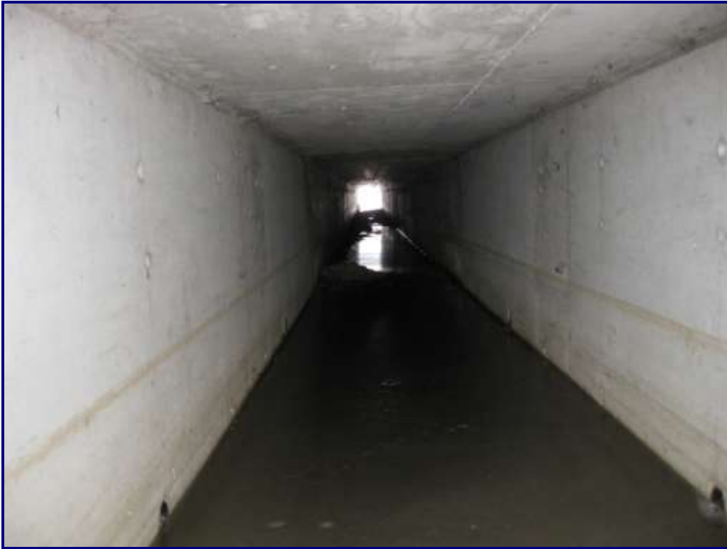
Photo 23 – Structure No. 4: Culvert Barrel
