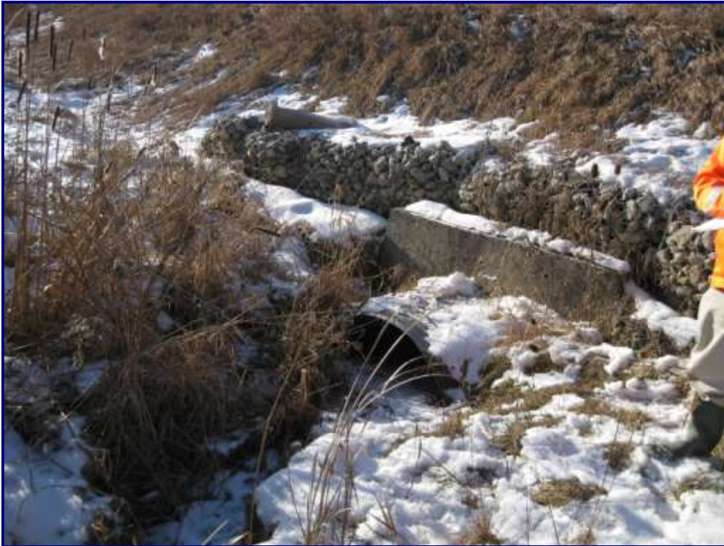
Photo 45 – Structure No. 11: South End of Culvert
