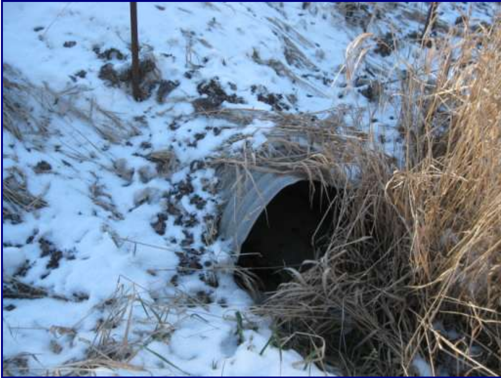
Photo 50 – Structure No. 12: East End of Culvert
