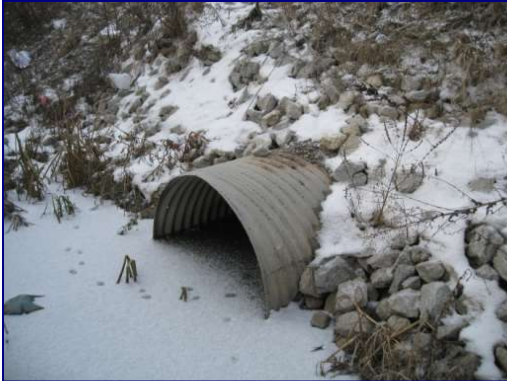
Photo 19 – Structure No. 3: South End of Structure
