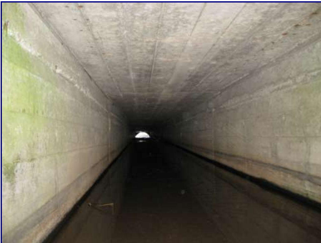
Photo 44 – Structure No. 11: North Barrel Looking South
