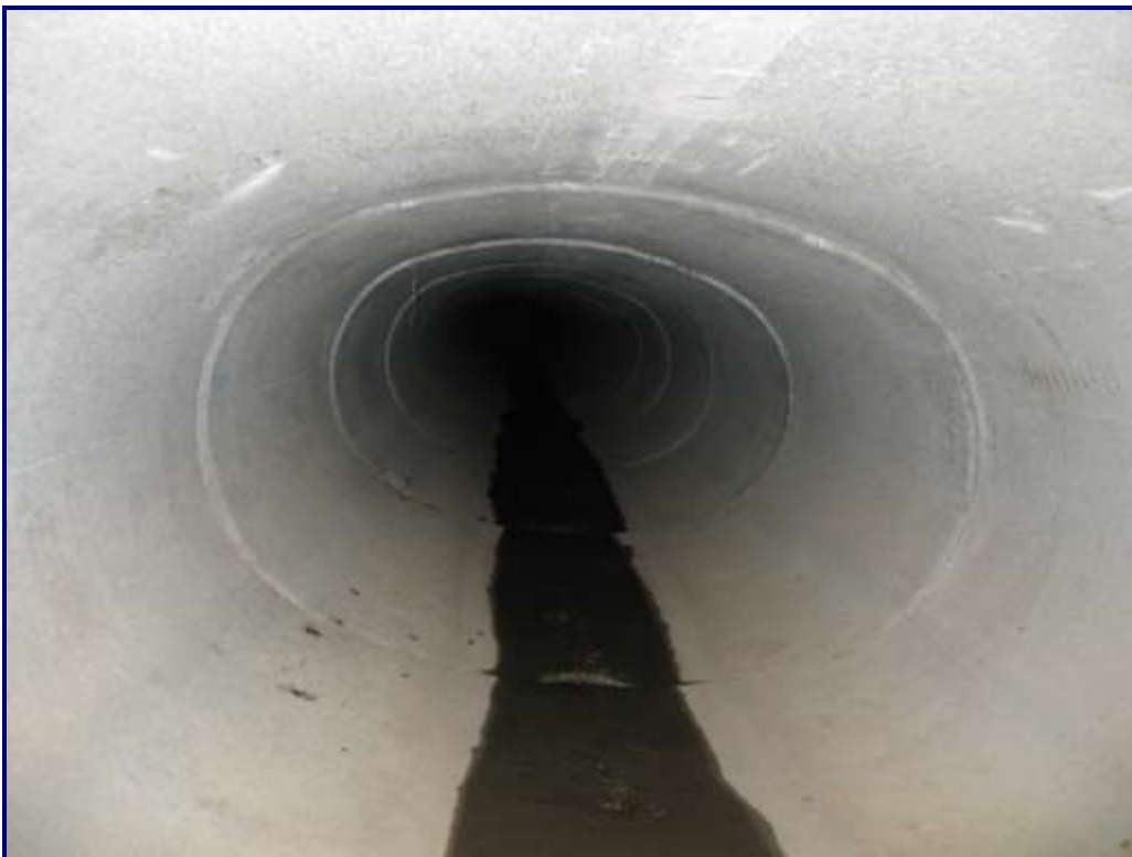
Photo 2 – Structure No. 1: Typical Culvert Barrel
