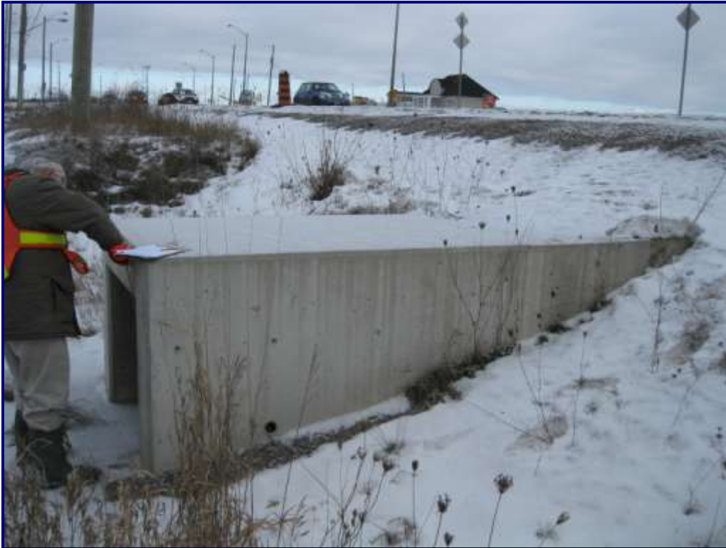
Photo 21 –Structure No. 4: North End of Culvert
