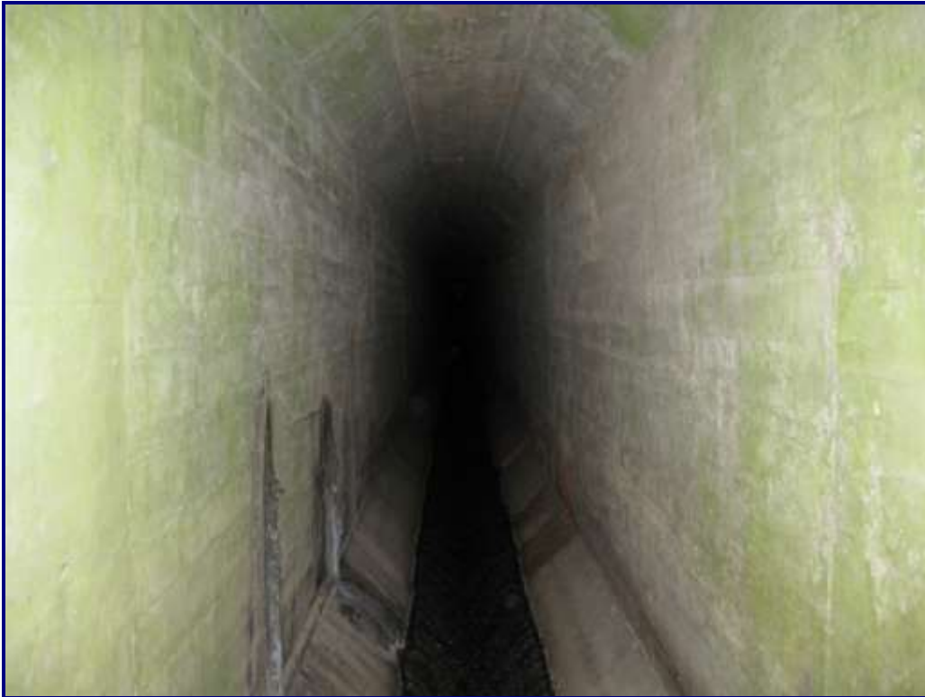
Photo 59 – Structure No.14: Culvert Barrel Looking North
