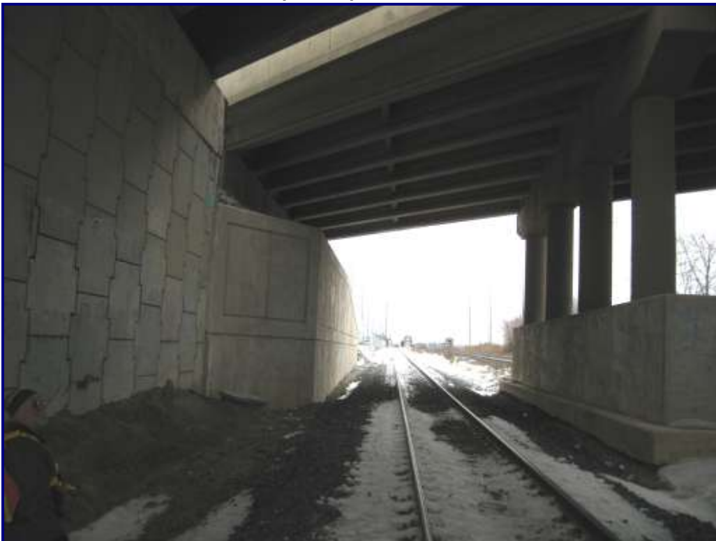
Photo 7 –Structure No. 2: Lead Track to Gold’s Layover Facility Protection Wall
