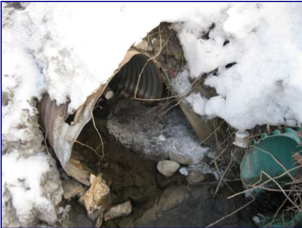
Photo 31 – Structure No. 8: West End of Culvert
