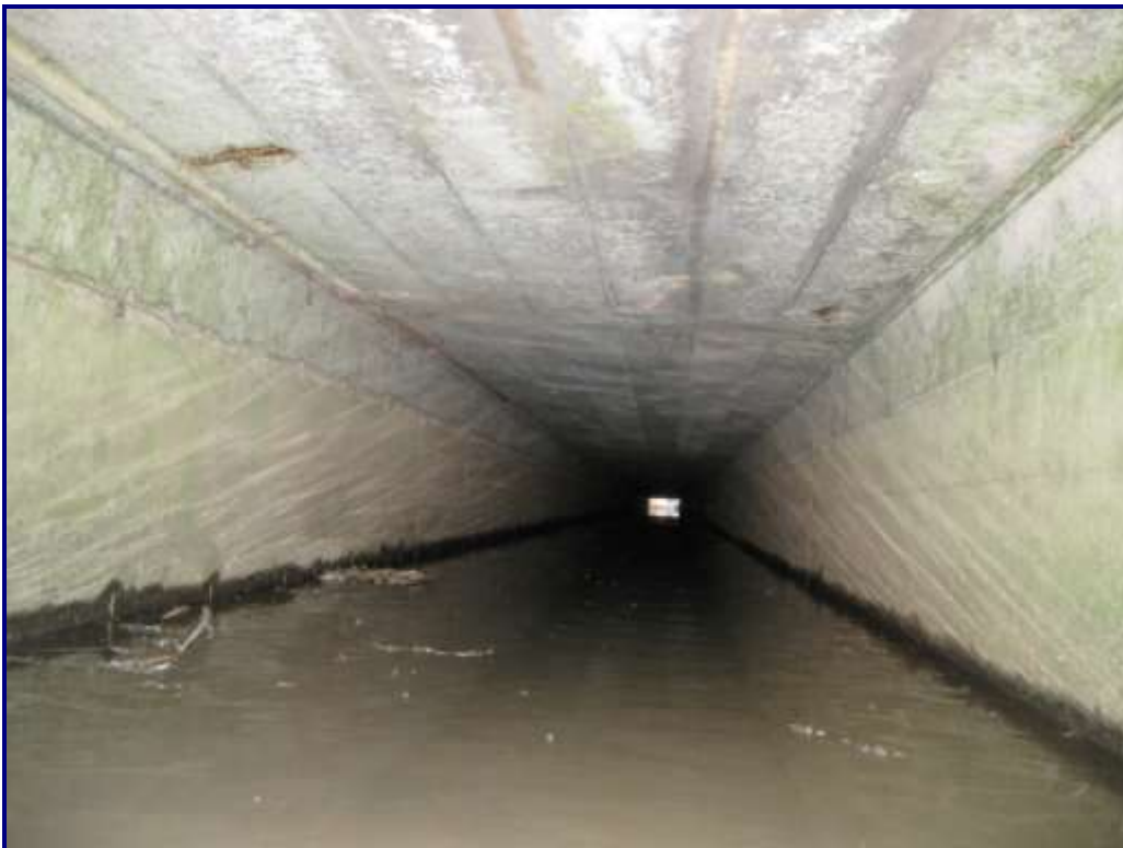
Photo 53 – Structure No. 13: North Barrel Looking South
