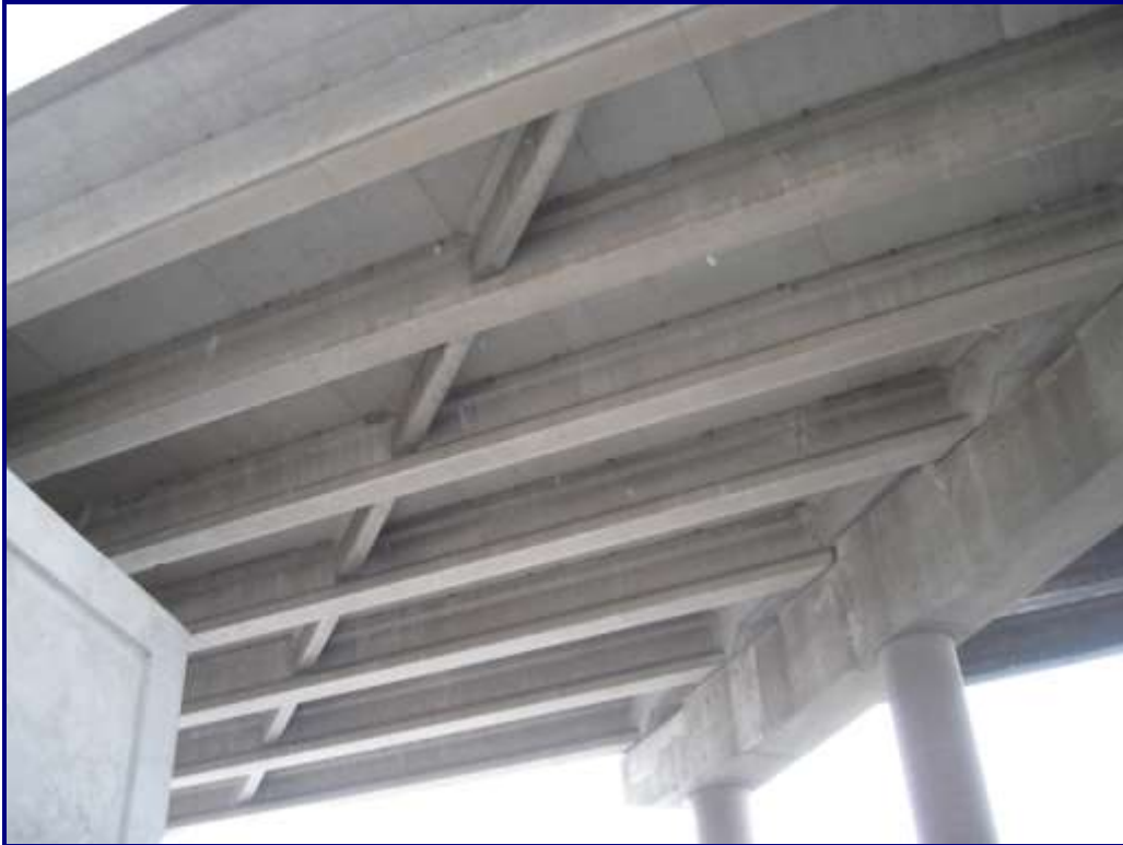
Photo 8 – Structure No. 2: Soffit
