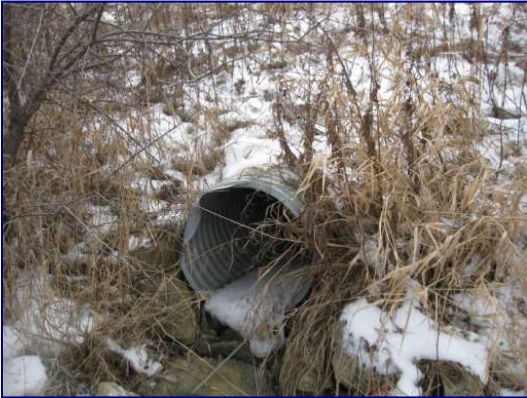
Photo 28 – Structure No. 6: East End of Culvert
