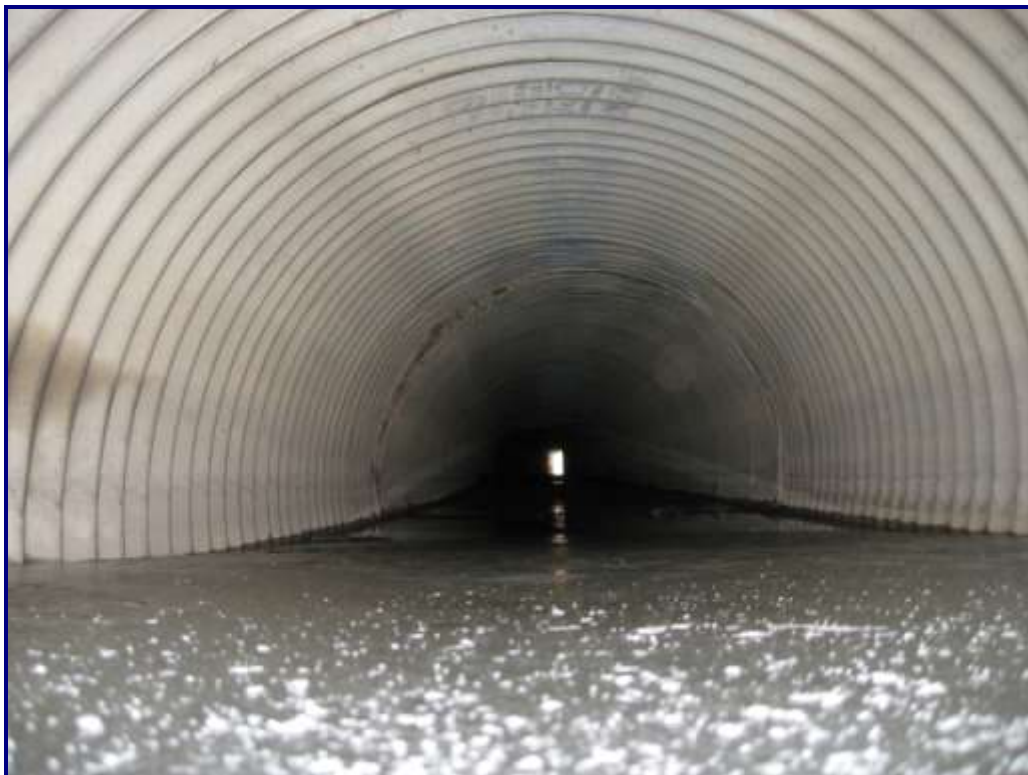
Photo 20 – Structure No. 3: South Barrel Looking North
