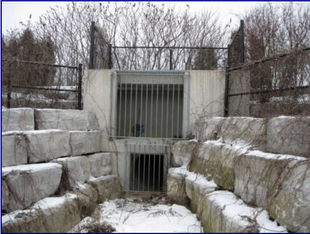
Photo 1 – Structure No. 1: Inlet Structure
