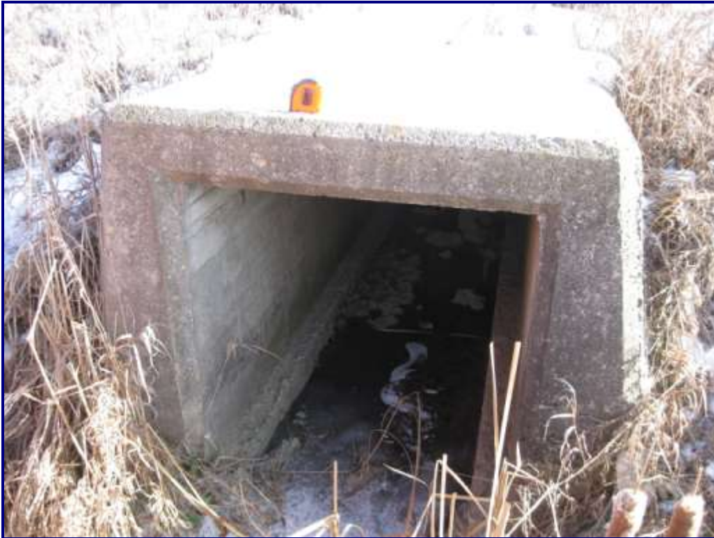
Photo 35 –Structure No.9: North End of Culvert
