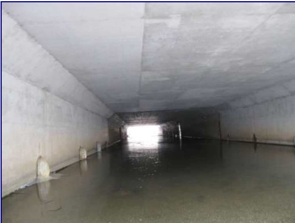
Photo 27 – Structure No. 5: South Barrel Looking North
