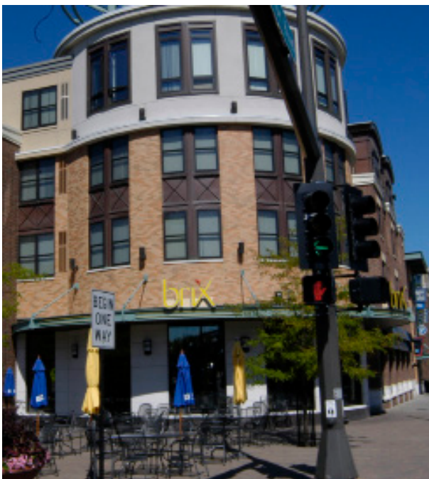
Above: At-grade retail is shown at the base of the building.
