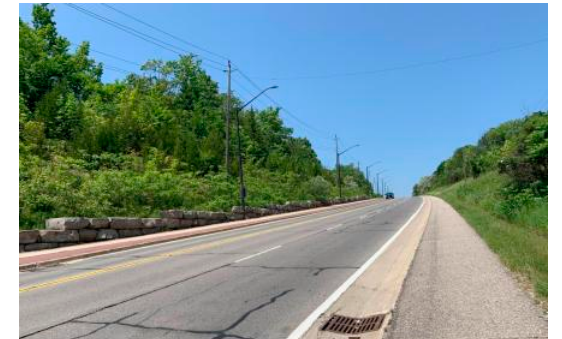
Storm Sews on Corridor Slope
