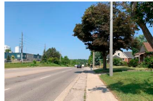
Pavement on Queen Street South
