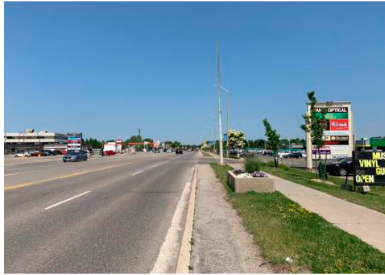
Queen St S: Consider raised median to limit left turns and avoid passing vehicles
