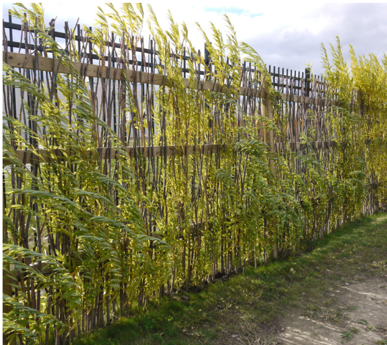
Streetsville GO Station Living Noise Attenuation Wall (Source: CVC)
