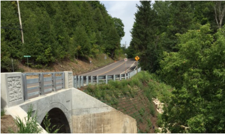
Belfountain Bridge Vegetated Retaining Wall. (Source: Region of Peel)
