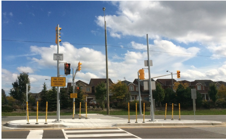
Pedestrian Crossing Island. (Source: Region of Peel)
