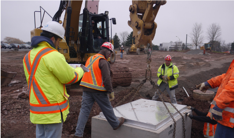
Installation of proprietary treatment device. (Source: Credit Valley Conservation)
