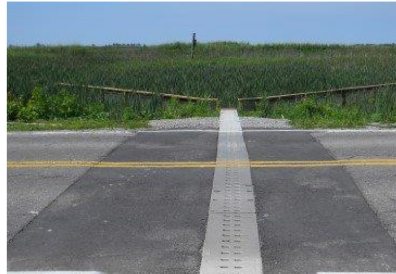
Turtle Passage Structure, Guelph, ON (Source: Chris Parent, Cole Engineering)
