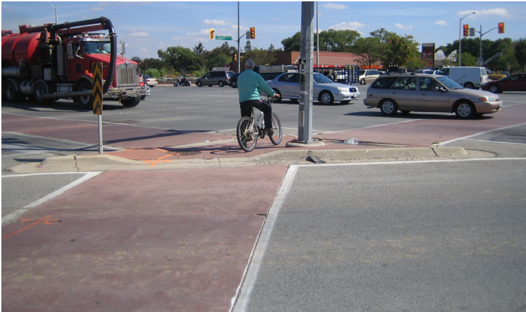
Bicycle crossing at Steeles and Hurontario (Source: Region of Peel)
