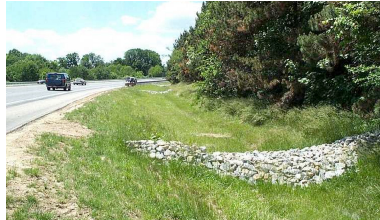
Enhanced Grass Swale Built with Riprap Check Dams (Source: Delaware Department of Transportation)
