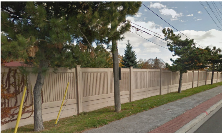
Pervious Concrete Sidewalk Along Dixie Road (Source: Region of Peel)
