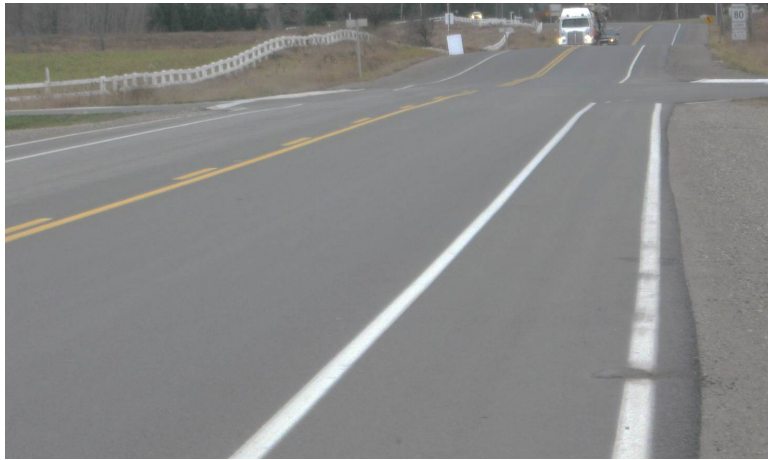
Paved Shoulder for Cycling on King St (Source: Region of Peel)
