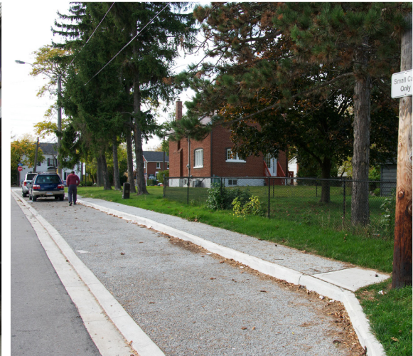
Pervious concrete lay-by parking in Streetsville. (Source: CVC)
