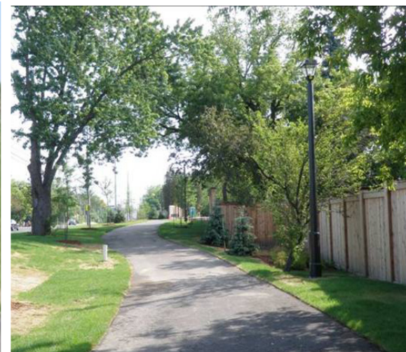
Wooden noise attenuation wall (Source: Region of Peel)
