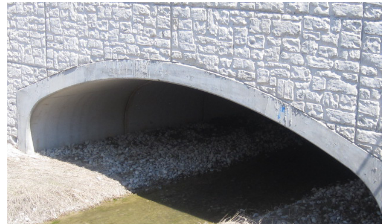
Enhanced culvert (Source: Region of Peel)
