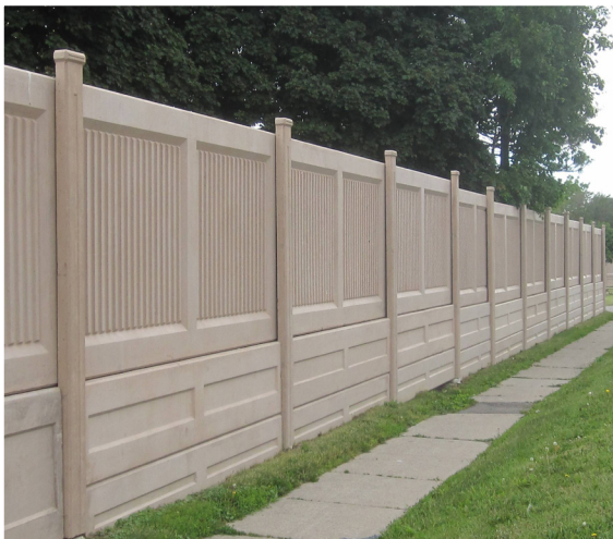
Concrete Noise Attenuation Wall, Dixie Road, Brampton (Source: Region of Peel)
