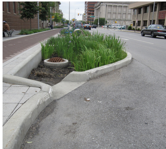
Bioretention Curb Extension (Source: Credit Valley Conservation)
