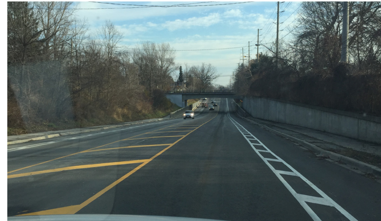
On-street Bicycle Lane with a 0.5m Buffer on Dixie Road (Source: Region of Peel)
