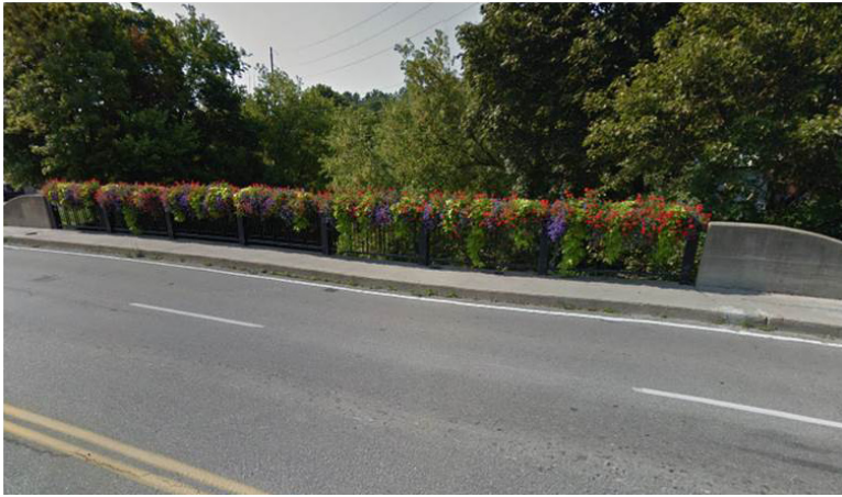
Heritage Bridge in Bolton Enhanced with Hanging Baskets. (Source: Region of Peel)
