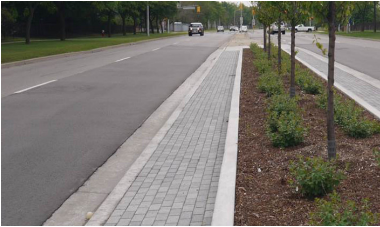
Green Infrastructure Installation within Median (Source: Credit Valley Conservation)
